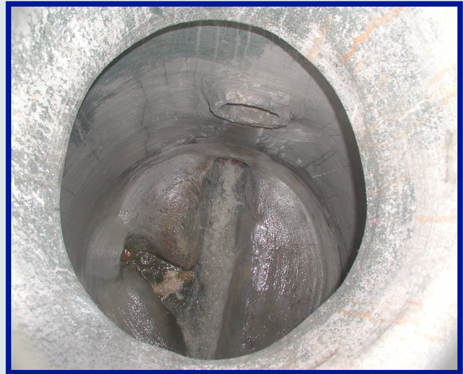
After Cementitious Rehabilitation
