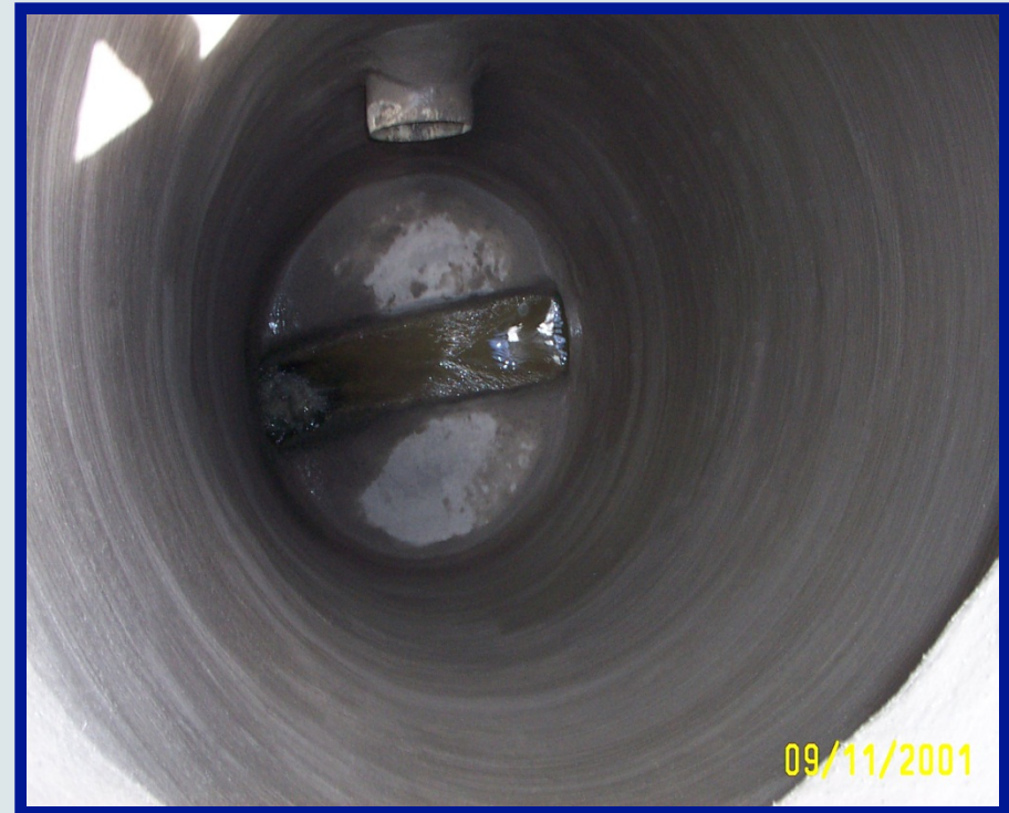
Existing Coating Removed and Mortar Installed
