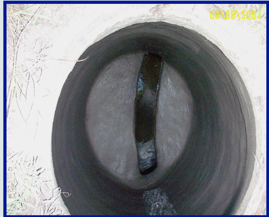
Rehabilitated Entirely with Cementitious Mortar
