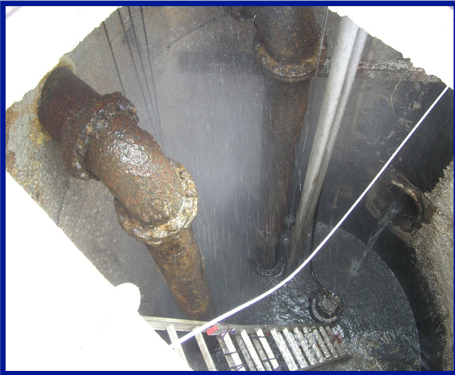
Existing Wet Well
