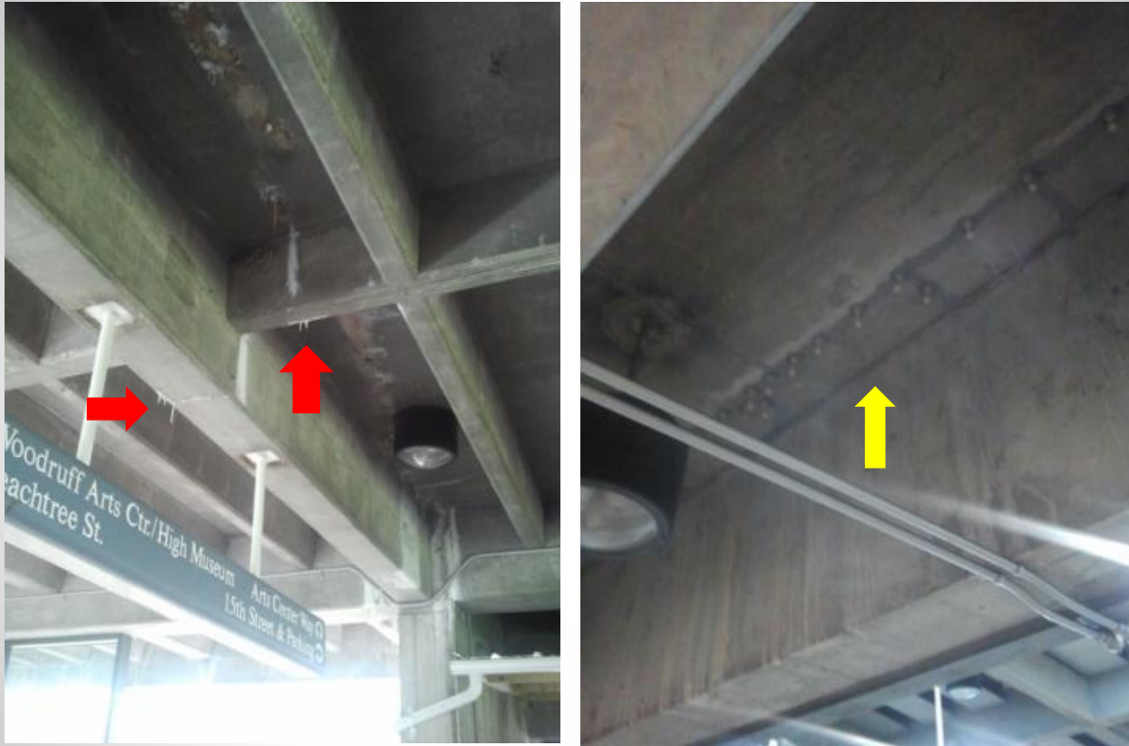
Arts Center Station – MARTA Atlanta, Georgia
