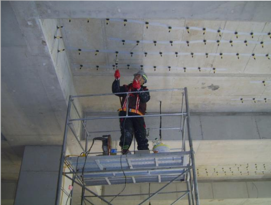
Parking Deck Overhead Crack Repair
