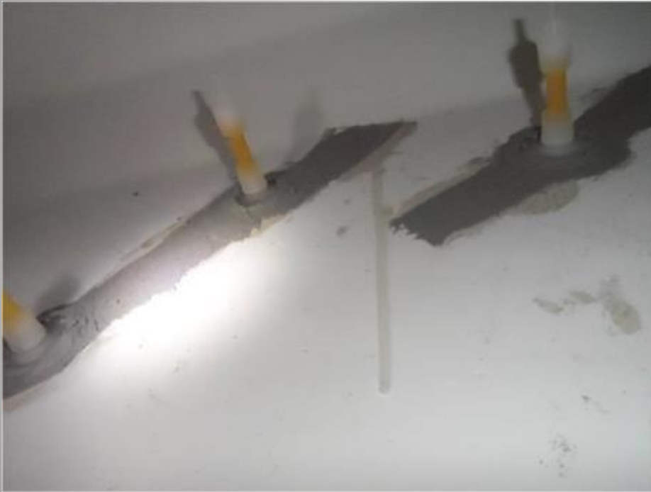
Double Tee Stem Repair Atlanta, Georgia
