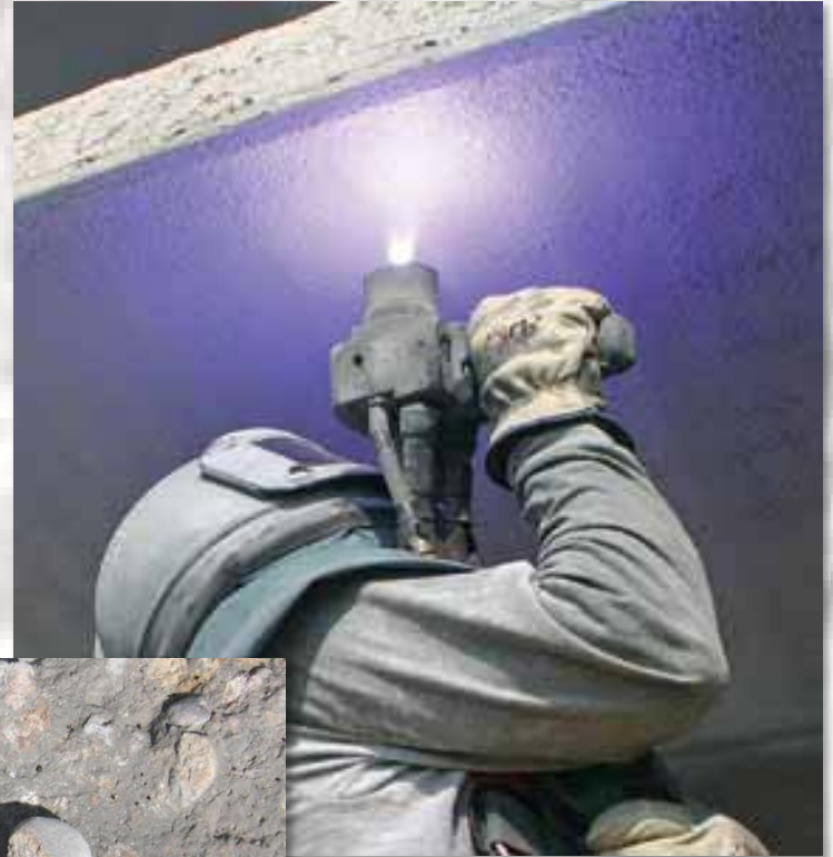
Spray Arc Metalizing
