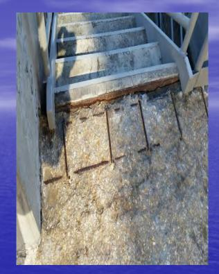
Fig. A & B: Surface cracks allow water into the concrete to cause further damage.
