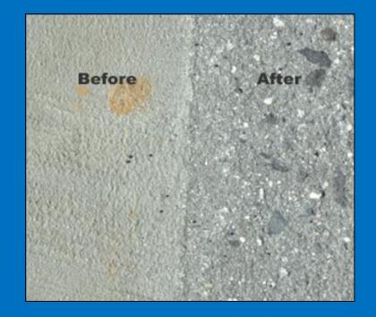
The quality of the substrate preparation determines the adhesive strength between the substrate and the installed system to prevent cohesive failure of the "vapor" barrier
