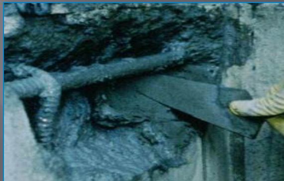
Installing Repair Mortar
