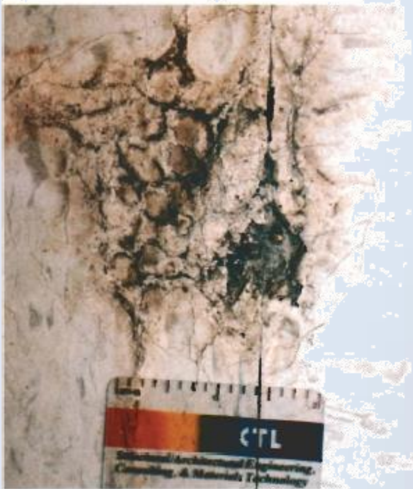
Figure 3-5. Vinyl composition tile (closeup, top) has been attacked and degraded by alkalis carried in moisture rising from below along a sawcut contraction joint in a retail store (arrows, bottom). (IMG15965, IMG16000)
