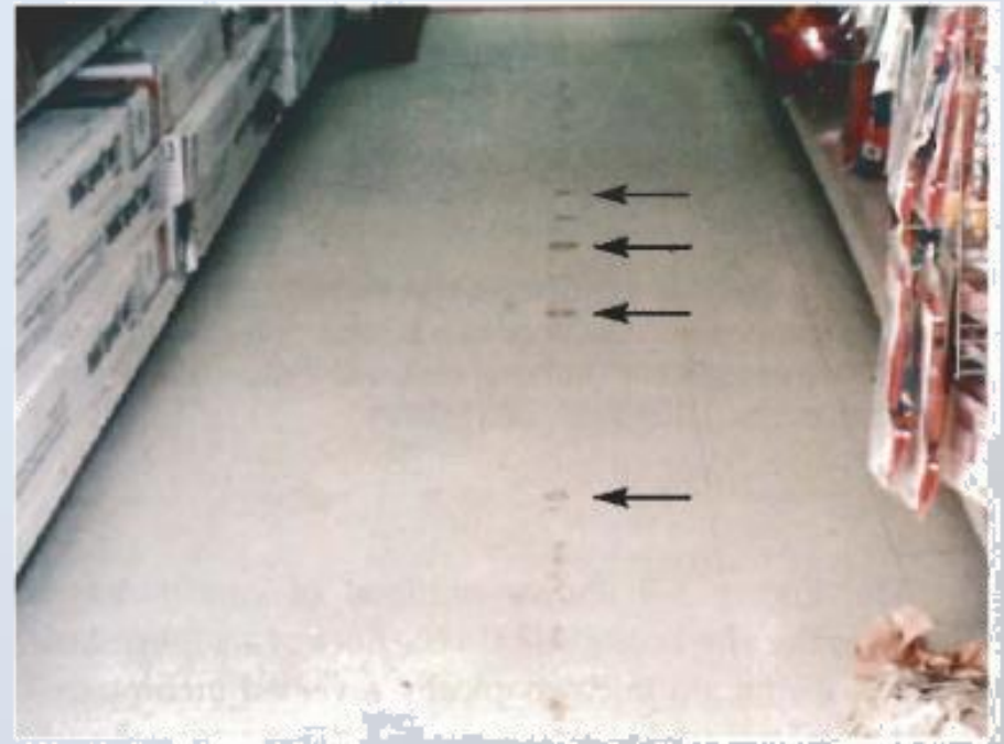
Figure 3-5. Vinyl composition tile (closeup, top) has been attacked and degraded by alkalis carried in moisture rising from below along a sawcut contraction joint in a retail store (arrows, bottom). (IMG15965, IMG16000)
