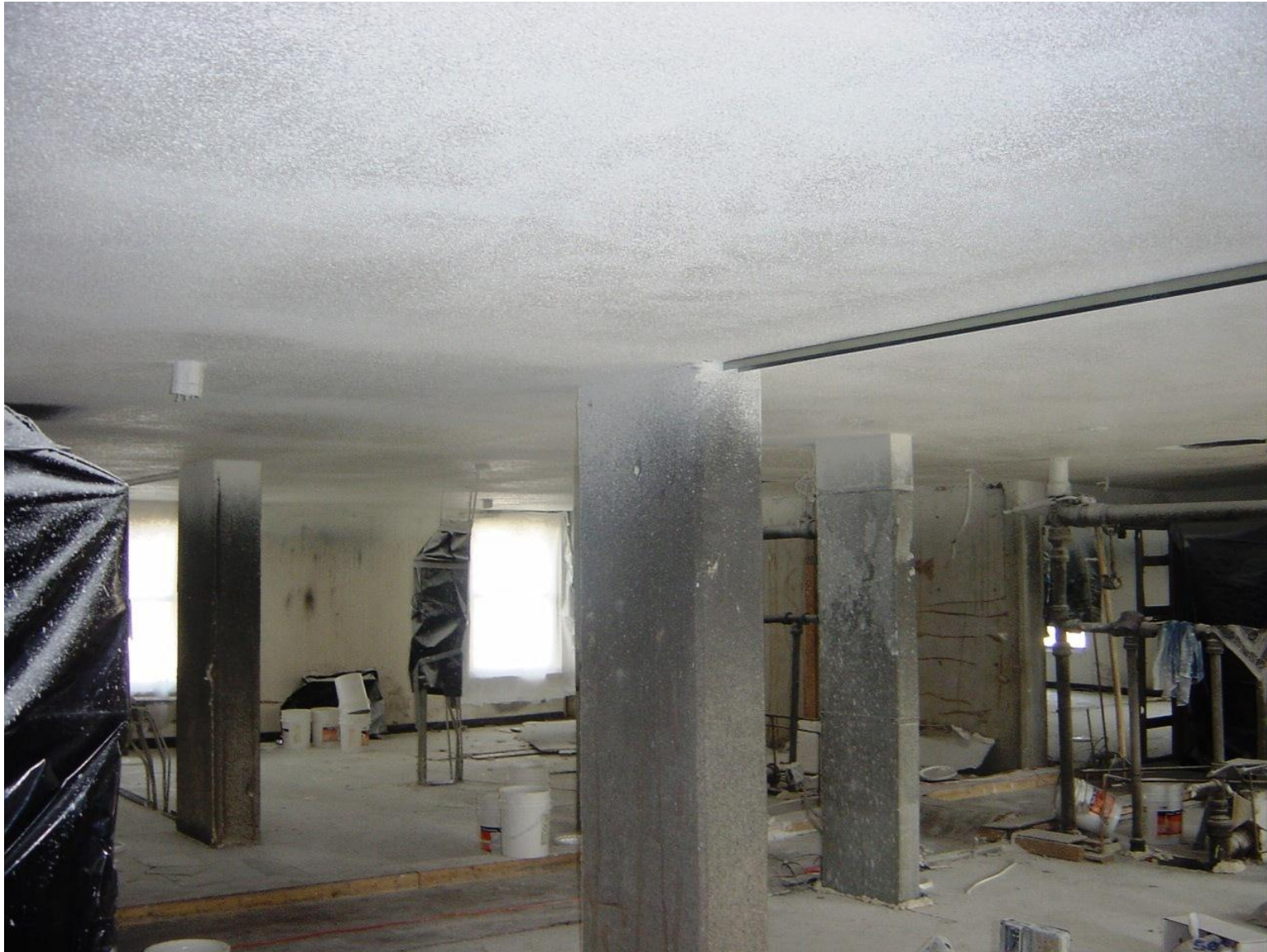
Overall of completed repair.
