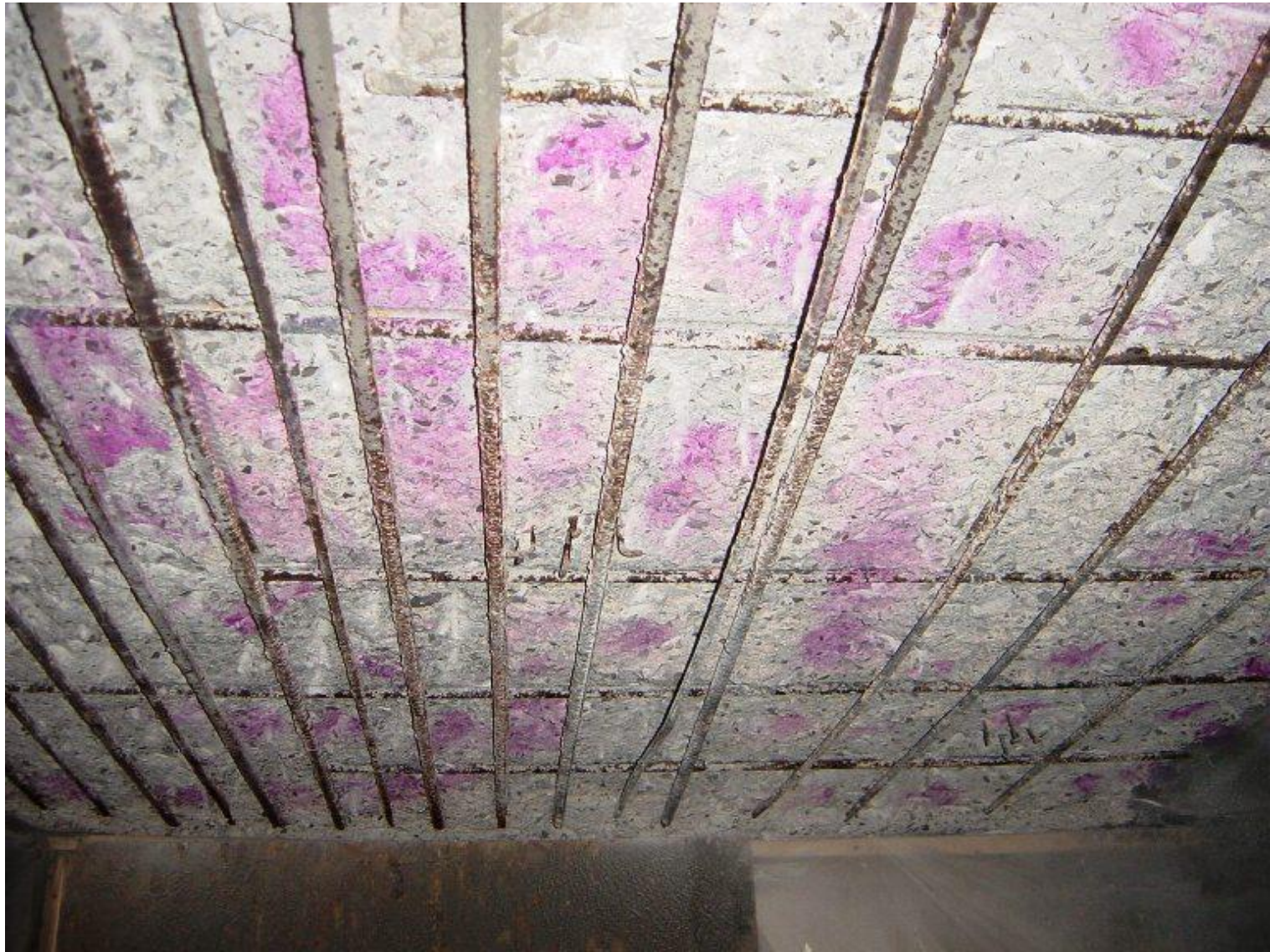
Carbonated concrete removed and carbonation checked with phenolphthalein.
