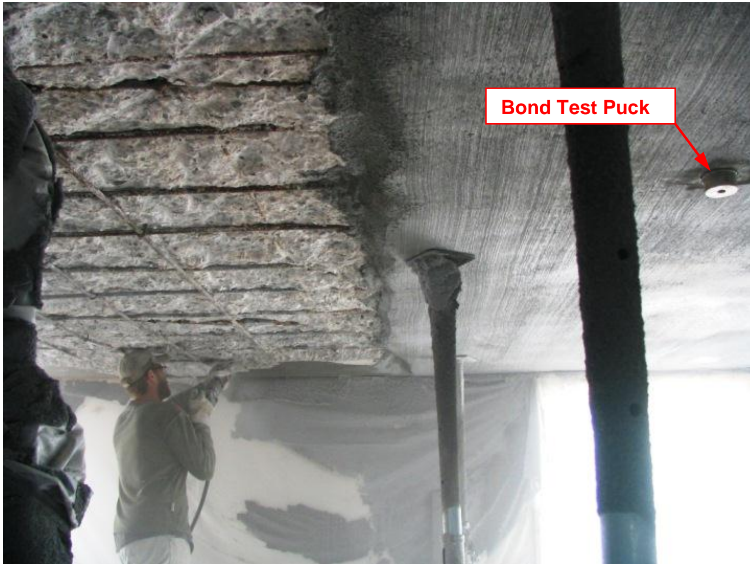
Removal of existing concrete along side completed shotcrete repair *POSTER*.
