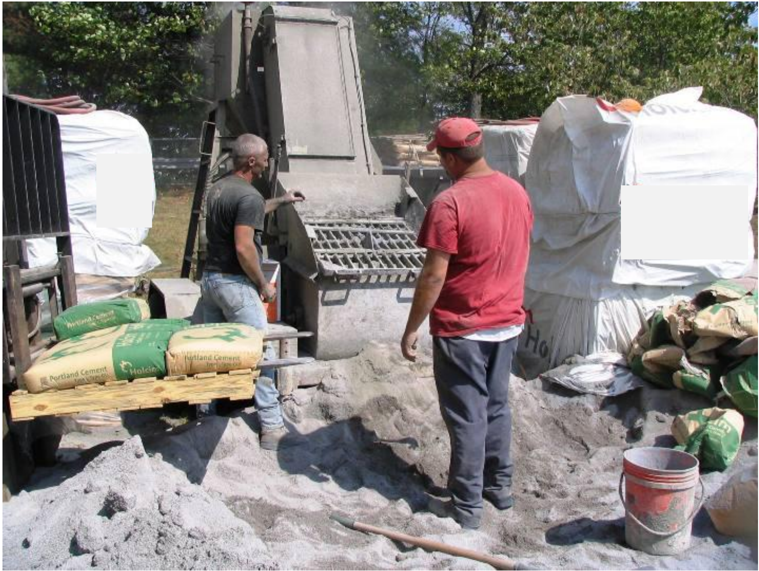
Mixing station outside facility.
