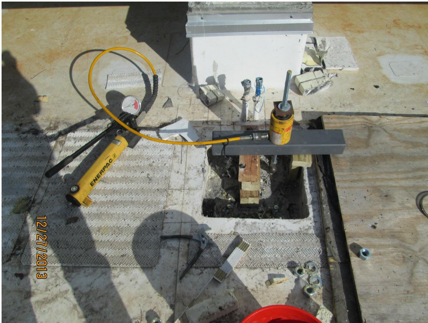
Adhesive Anchor and Safety Tie Back Testing
