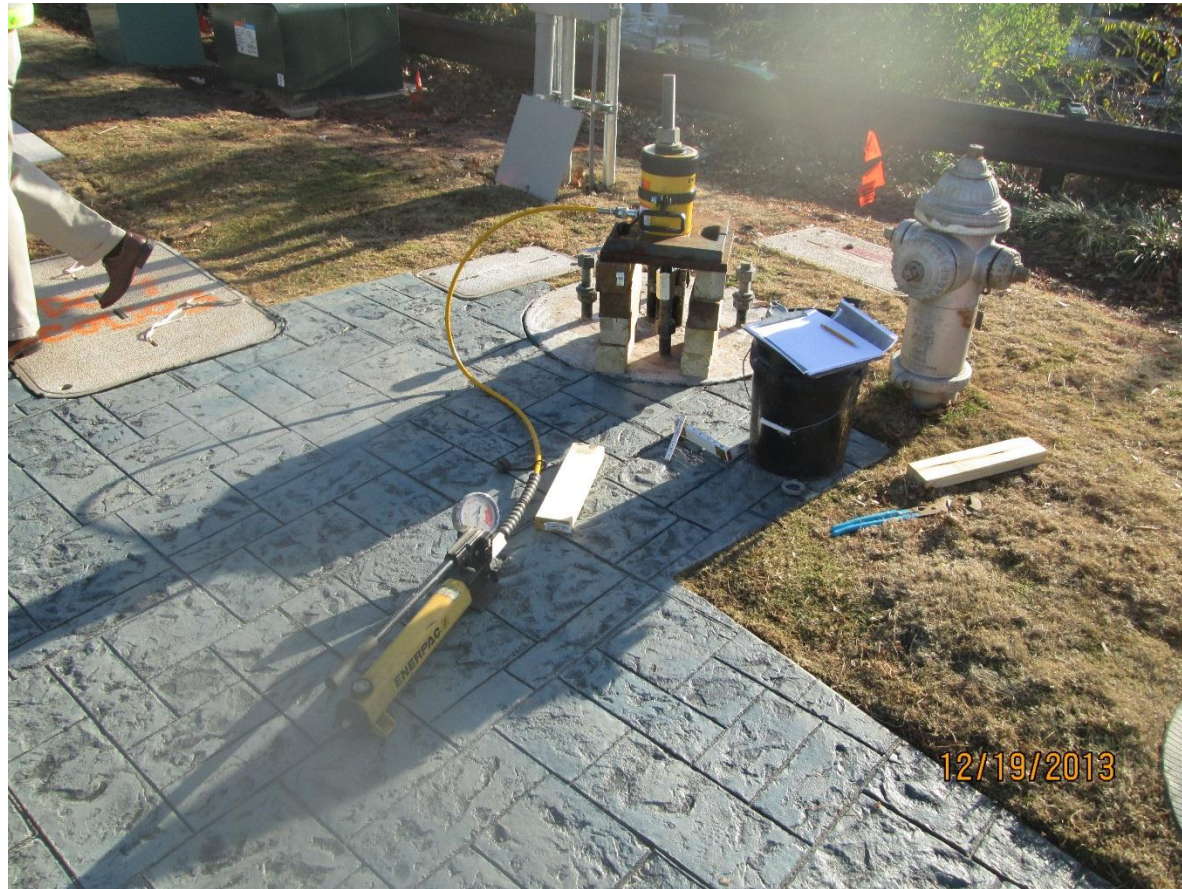
Proof Load Anchor Bolt Testing
