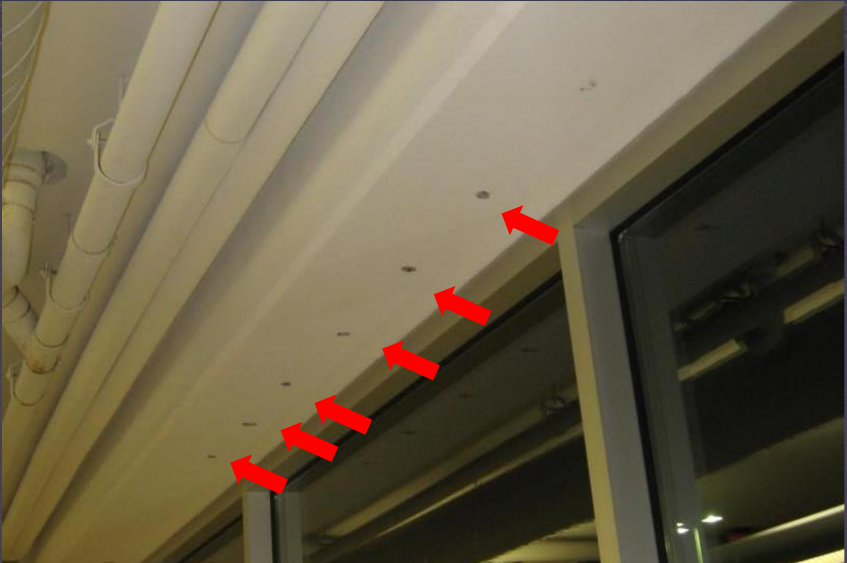
Dowels installed into underside of beam
