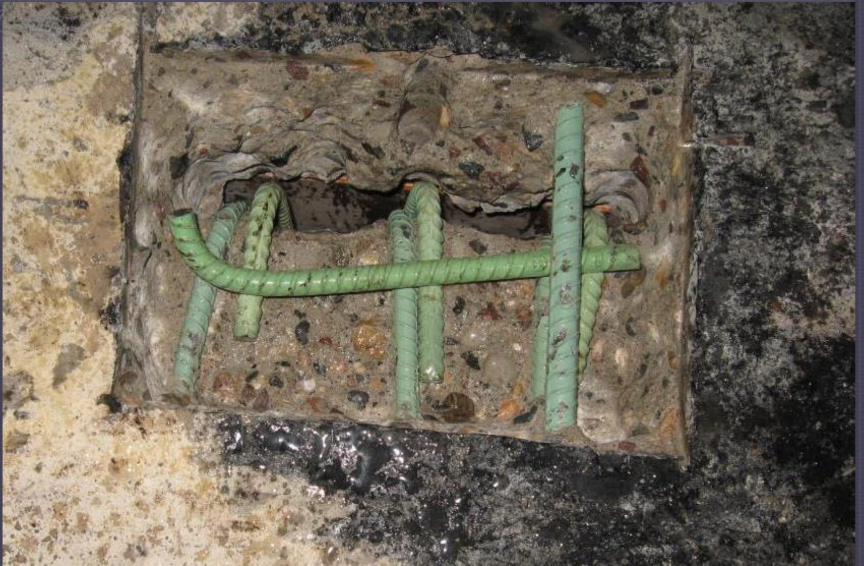
Hooked dowels installed in roof
