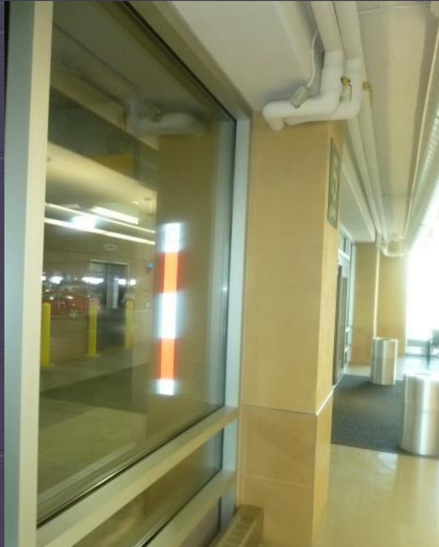
Typical beam in public lobby area
