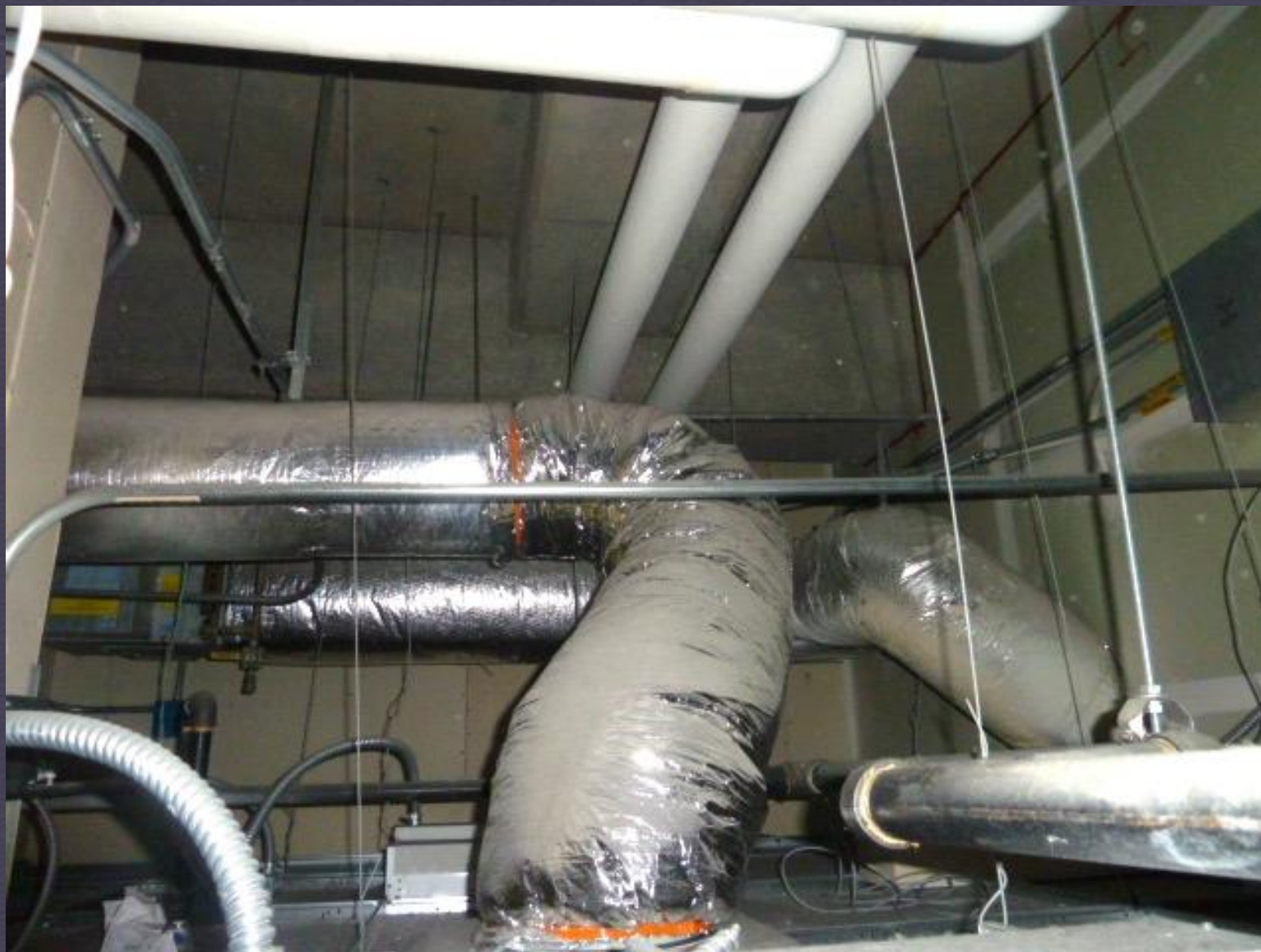
Congested areas below beams
