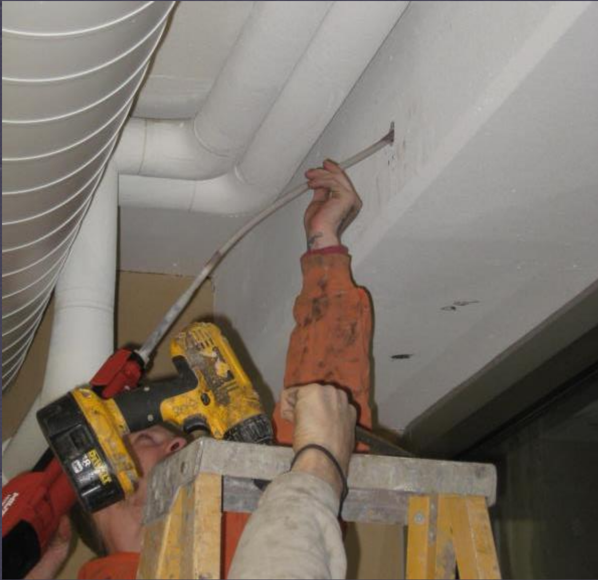
Epoxy fill of dowel hole
