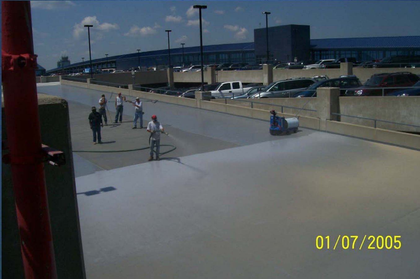
Top Coat Application
