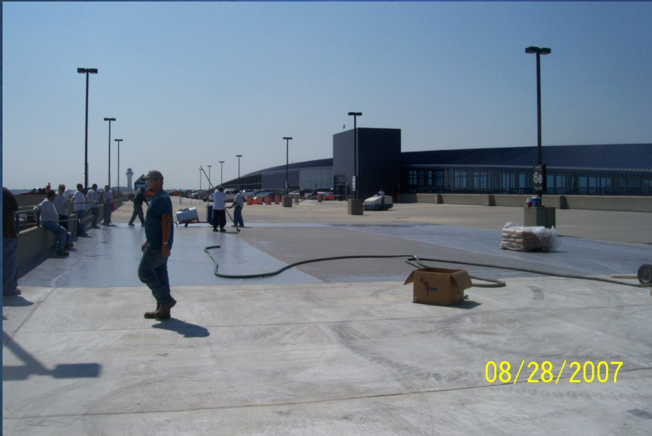
Base Coat Application
