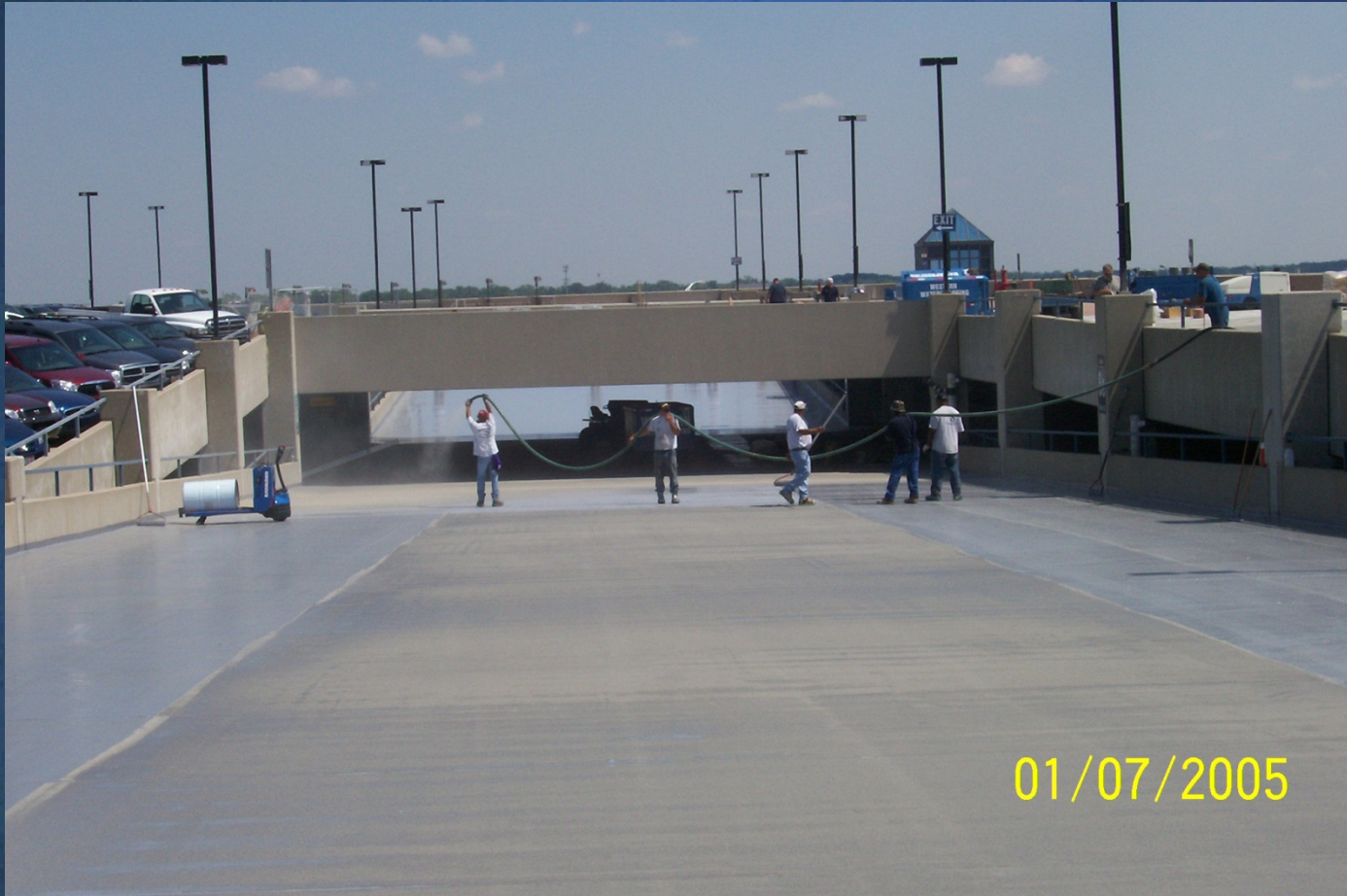
Traction Coat Application
