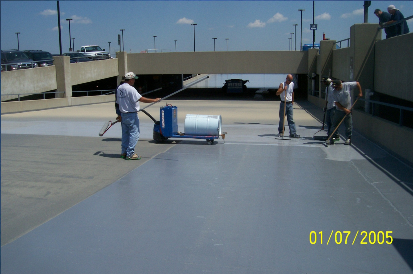
Top Coat Application
