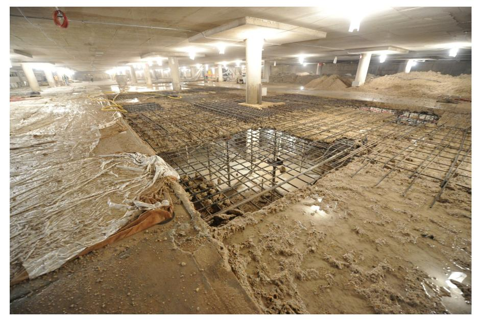
Installation of 47 tons of new reinforcing steel
