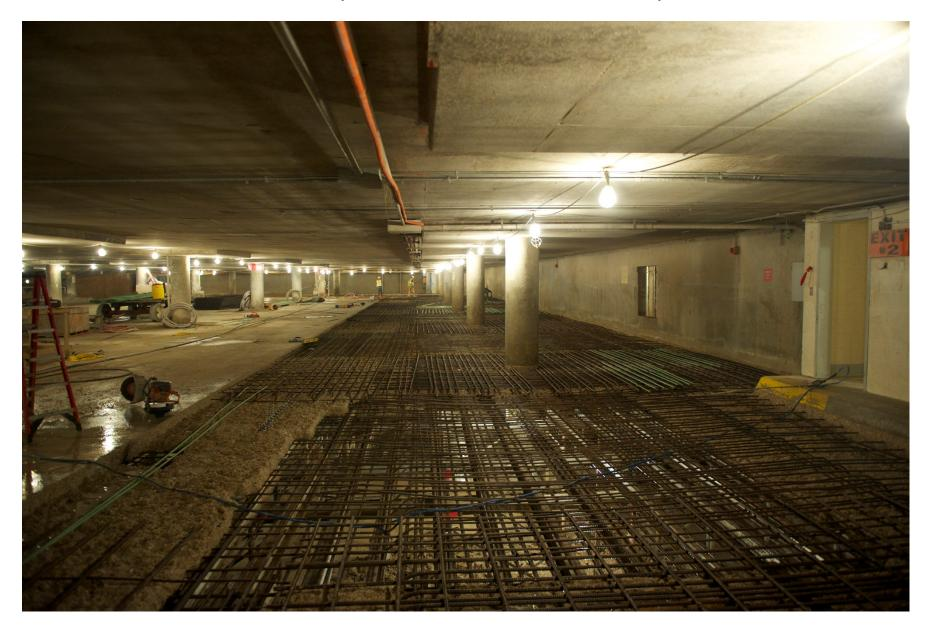
• 41,000 SF of 10" full depth slab repair
