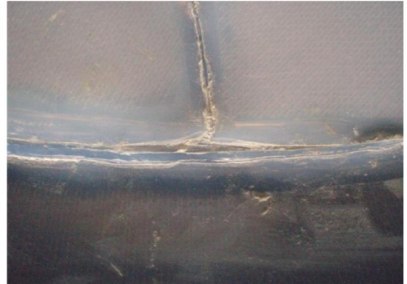
Lack of Fusion and Poor Fit
