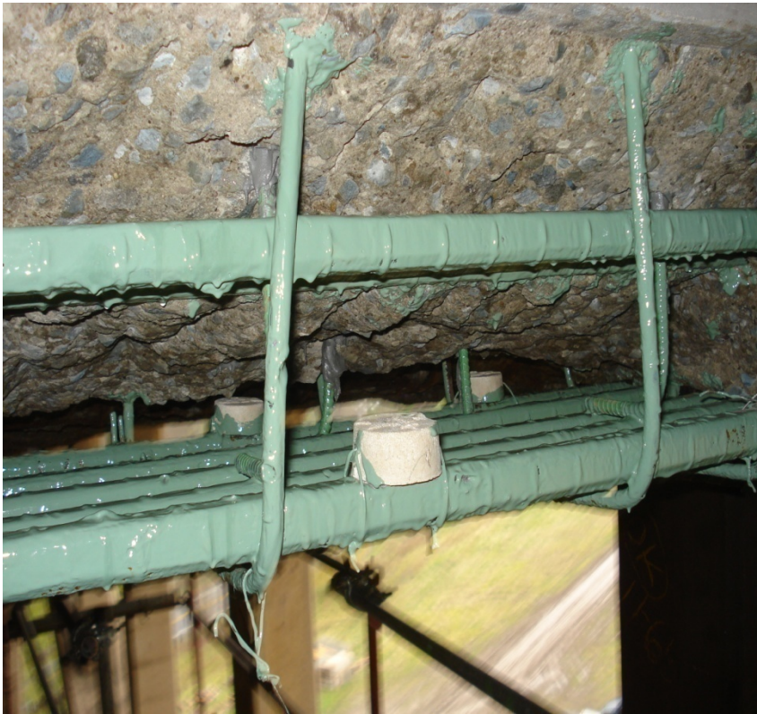
After cleaning/ Epoxy Coating Steel
