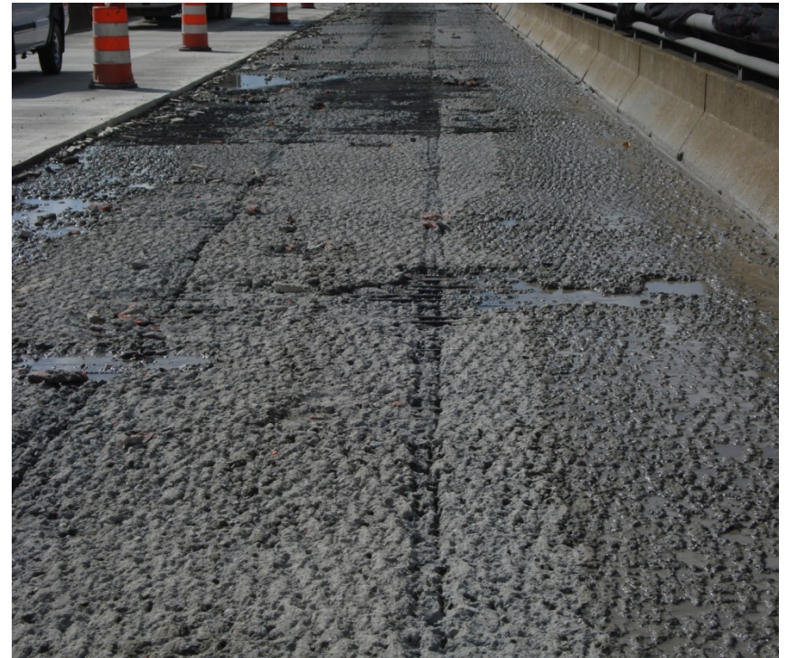
Hydro of Mt. Nebo Bridge
