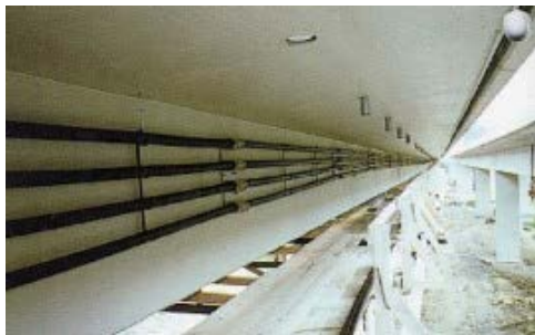
External Post-Tensioning
