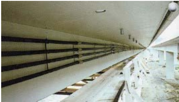
External Post-Tensioning
