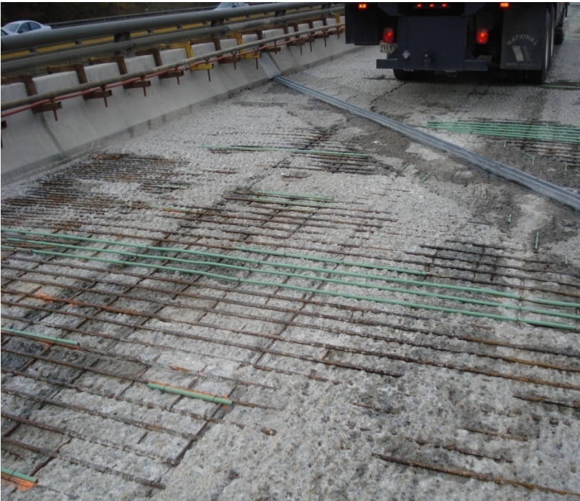
Glenfield Deck After Hydro
