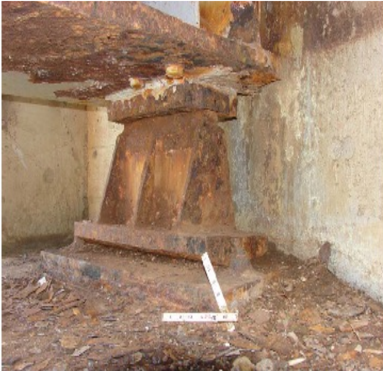
PHOTO 46 DIRT AND DEBRIS ON BRIDGE SEAT AND HEAVY CORROSION AND RUST ON EXPANSION BEARING MEMBERS AT NORTH ABUTMENT
