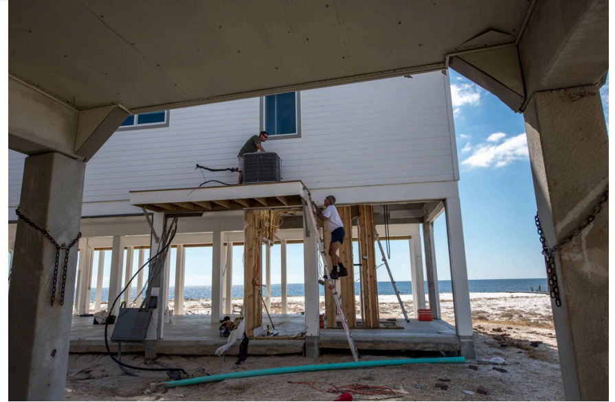
Rebuilding tear-away staircase Johnny Milano for NY Times, 2018
