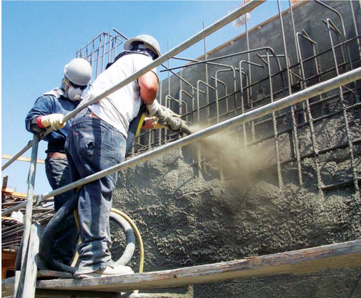
Traditional Shotcrete Repair
