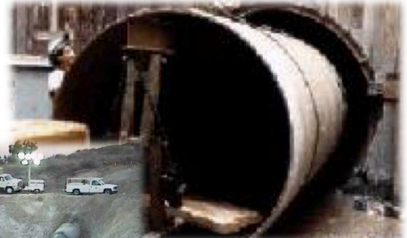
Dig up and repair (slipline)
