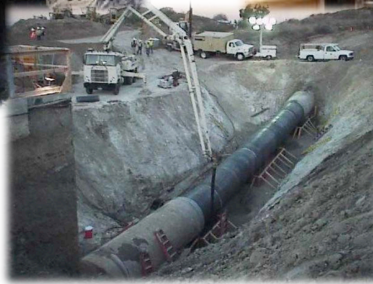
Dig up and replace
