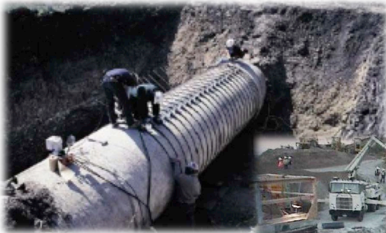
Post-tension repair
