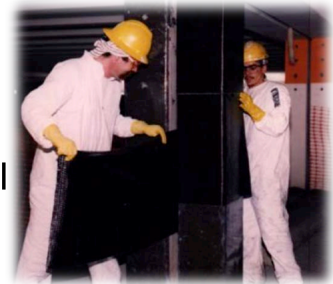
Retrofit of a Column
