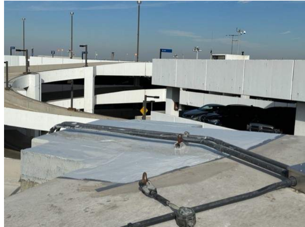
After installation of waterproofing membrane
