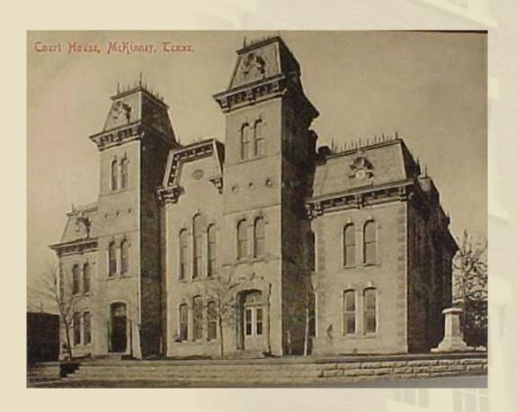
Unreinforced cut stone with limestone rubble infill
