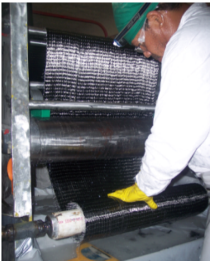
(4) Impregnate Carbon Fabric
