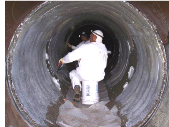
(3) Apply Tack Coat and Thickened Epoxy
