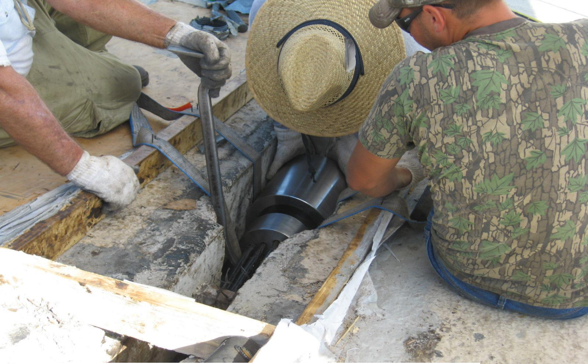
Installation of the New Coupling
