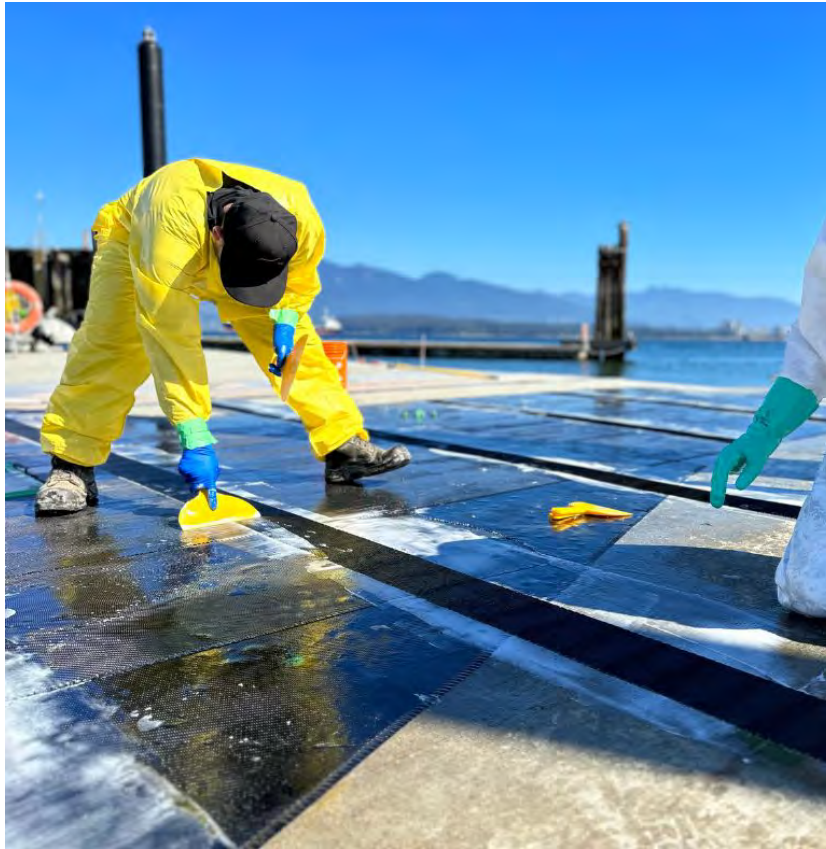
Crack Reinforcement and Structural Strengthening
