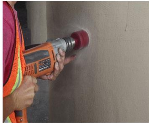
(a) Core drilling
