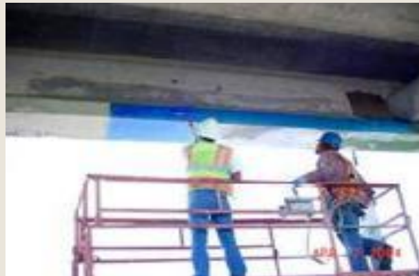
1 st Layer of FRP
