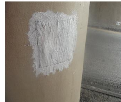
(f) Repaired surface
