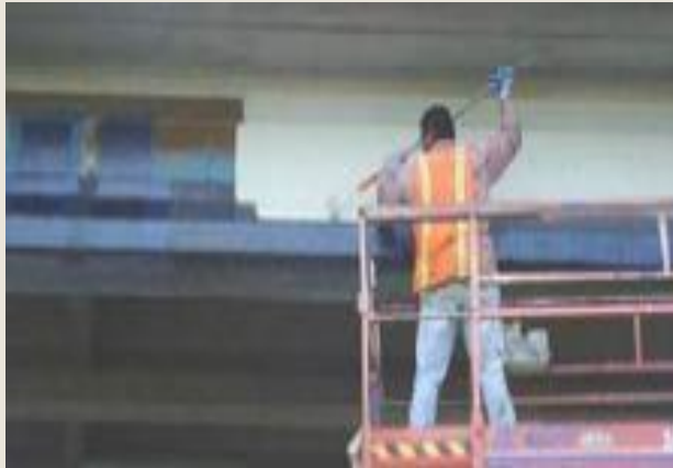
Top coat Application
