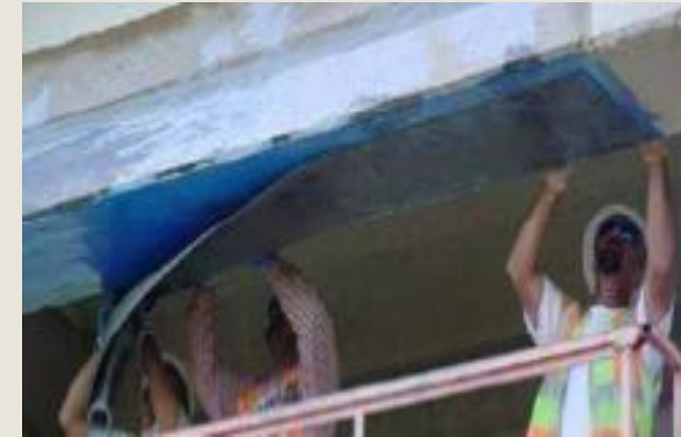
2 nd Layer of FRP
