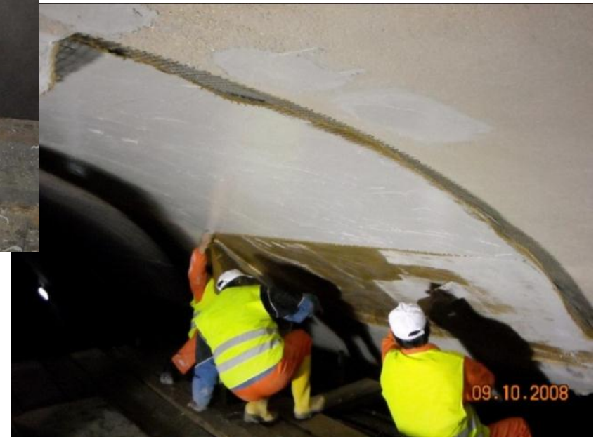
Application of FRCM at top portion of tunnel lining
