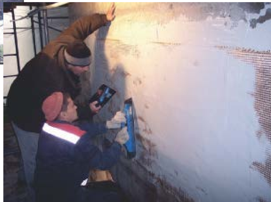
Workers trowel top finish over FRCM network within a heated tent
