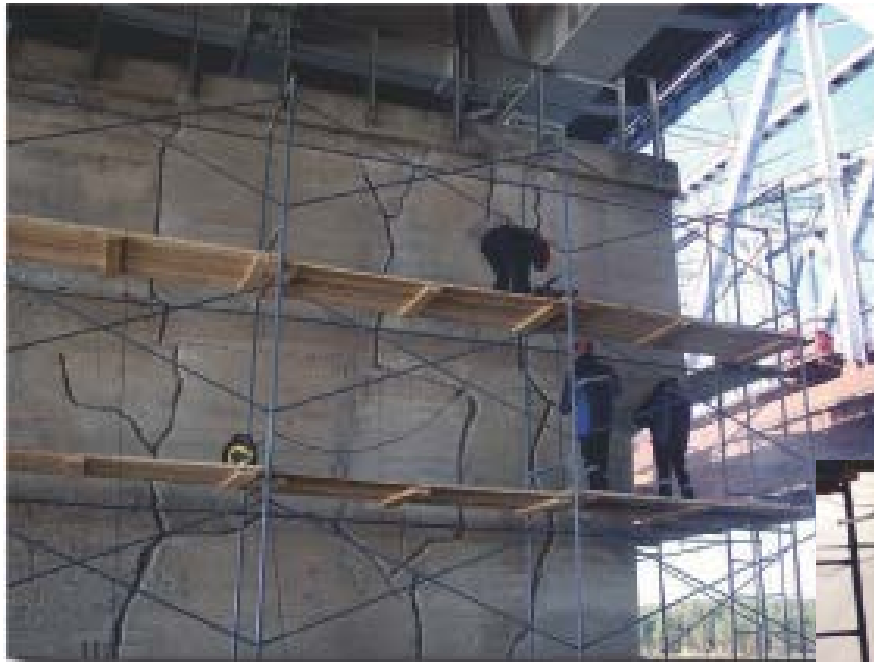
Workers repoint cracks prior to application of FRCM strengthening
