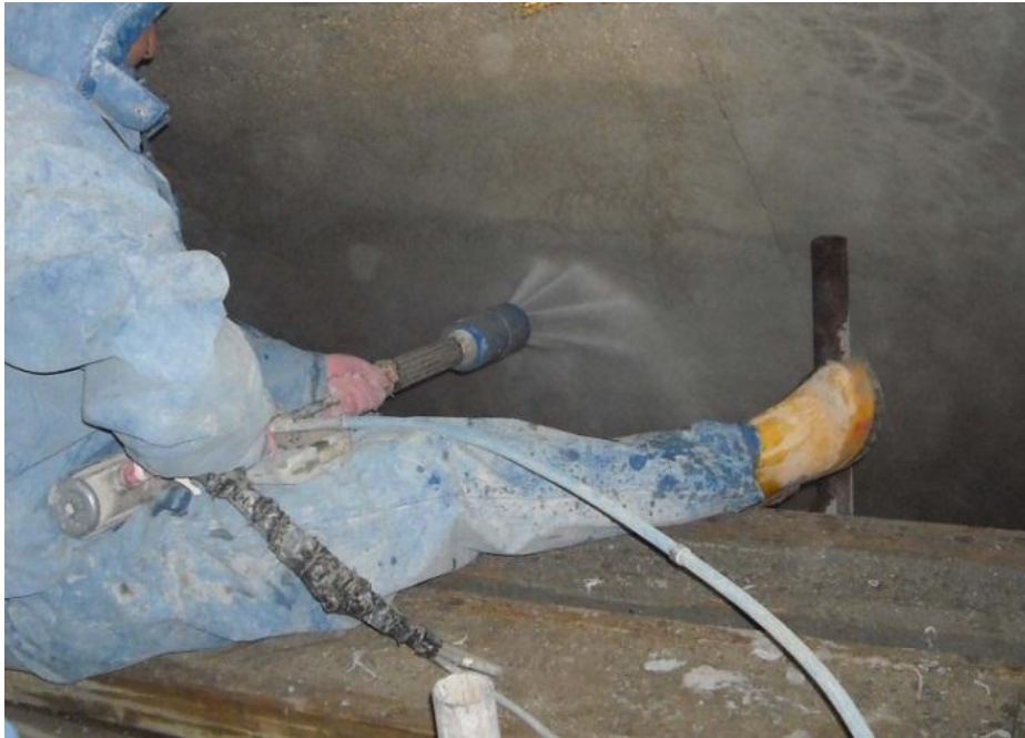
Surface preparation by hydrojetting
