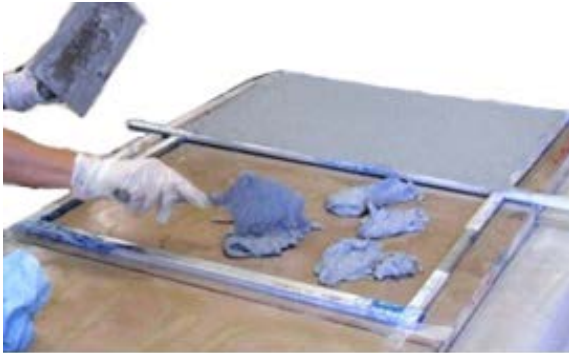
First layer of mortar
