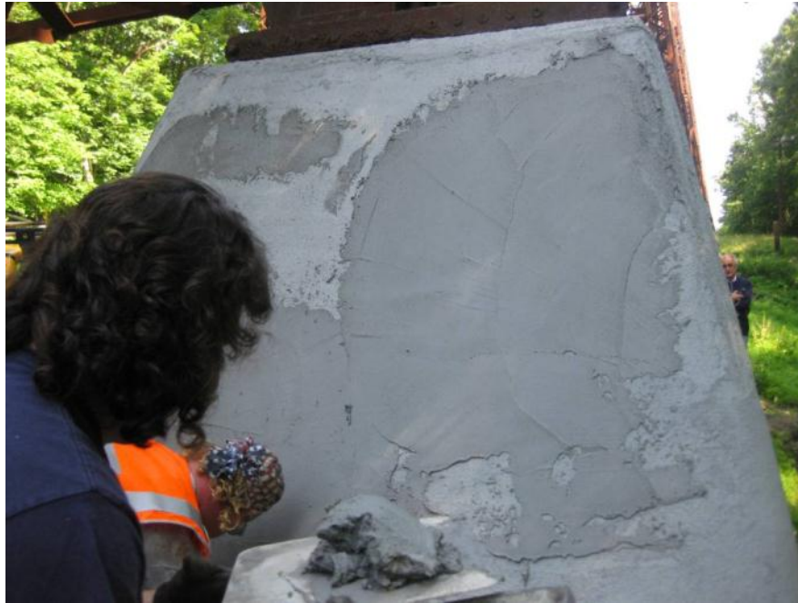
Worker patches the substrate
