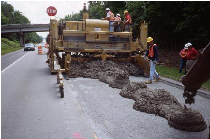
4-in bonded overlay placed on I85 in 1995 2-in bonded overlay placed on I295 in 1995
