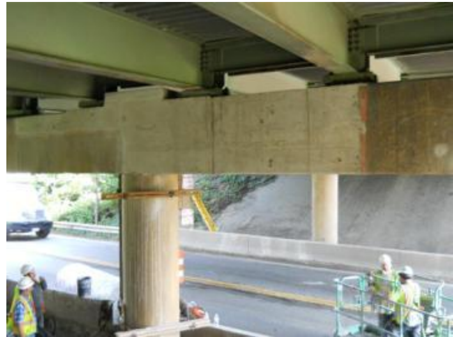
Completed pier cap
