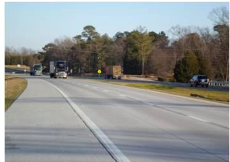
US 58 4-in bonded overlay and 7-in unbonded overlay placed in 2012 24
