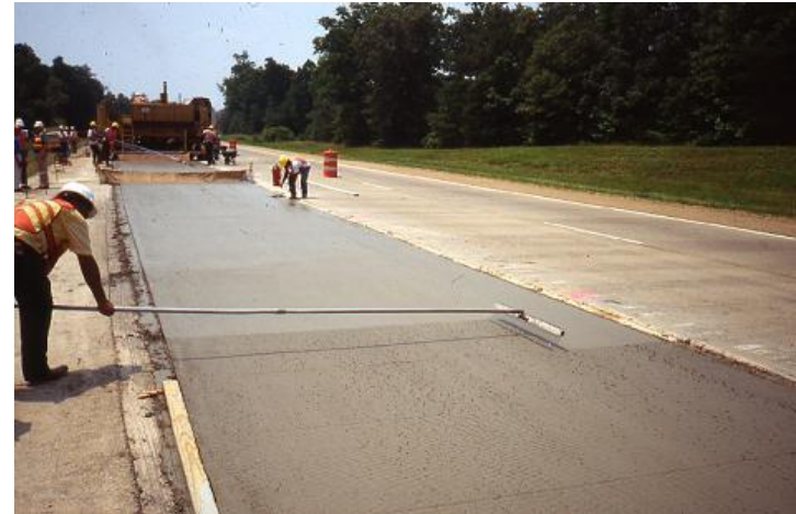
4-in bonded overlay placed on I85 in 1995 2-in bonded overlay placed on I295 in 1995
