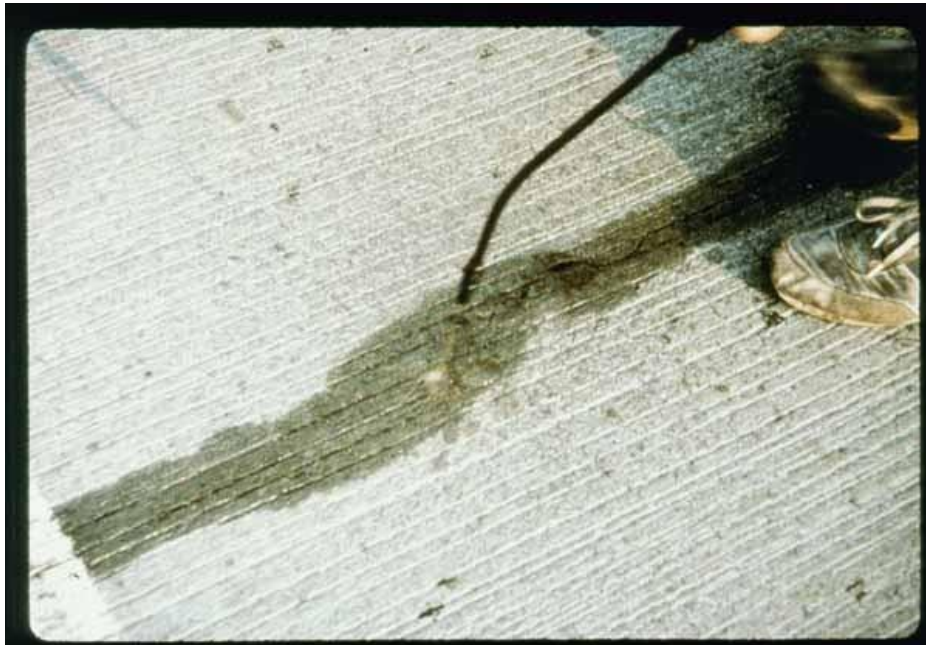
Individual Crack Application
