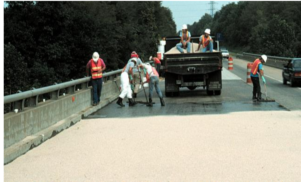
Placing epoxy prior to broadcasting aggregate
