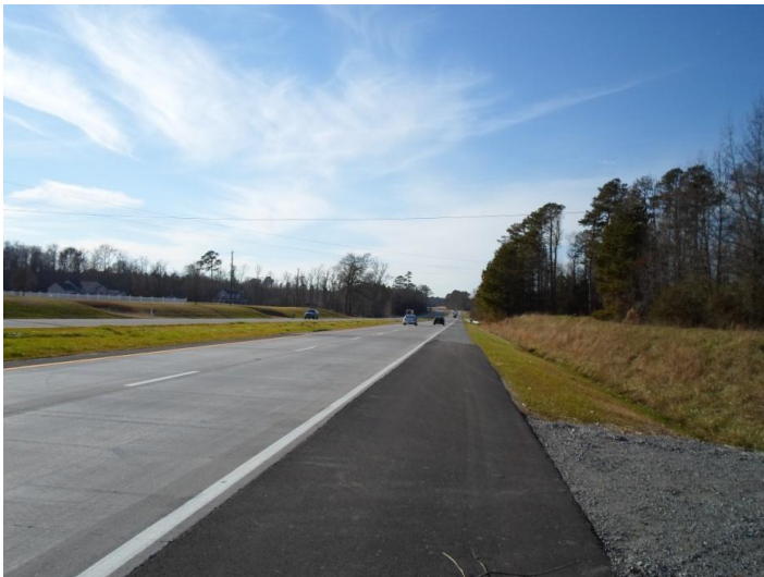
US 58 4-in bonded overlay and 7-in unbonded overlay placed in 2012 24
