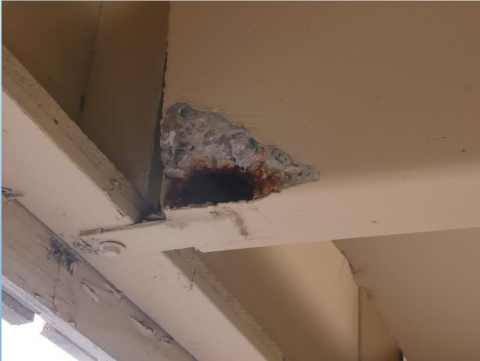
Concrete Spall
