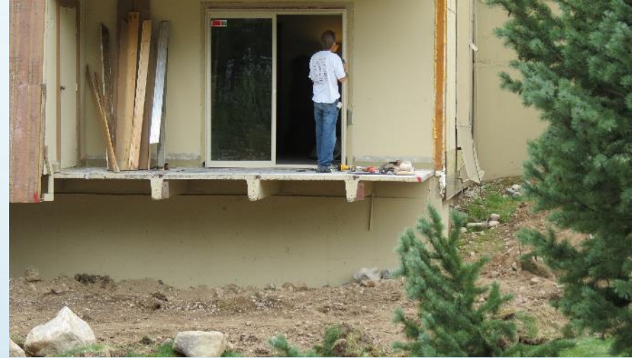
New energy efficient doors installed
