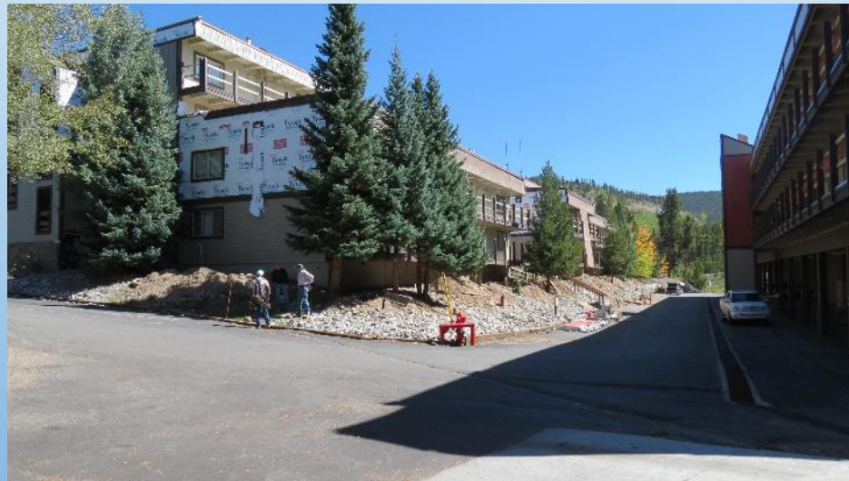
Upgraded insulation and building wrap
