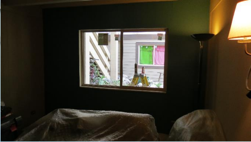
New energy efficient windows installed
