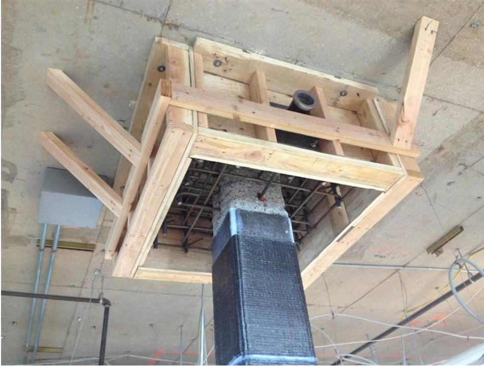
Shear Cap for punching shear deficiency
