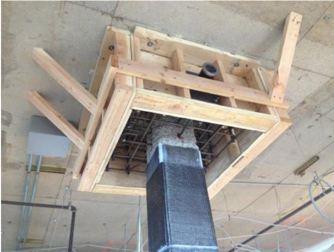
Typical 4-Sided Shear Cap
