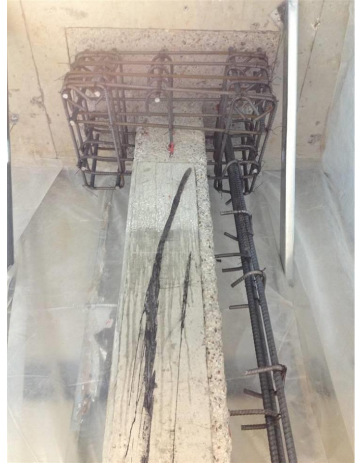
Shear Cap for punching shear deficiency
