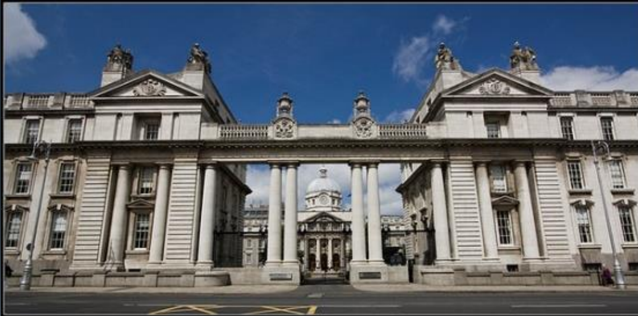
Colonnade, Prime Minister's Residence, Dublin, Ireland 1990 Installation 2012 system still performing
