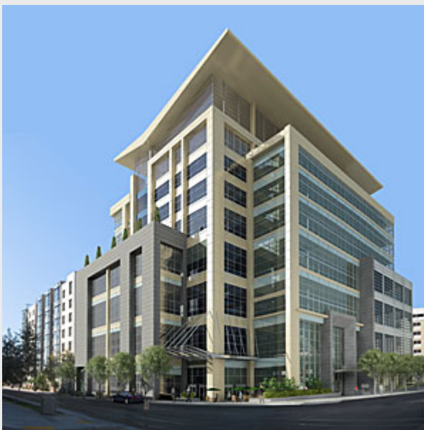
University classroom building located in downtown San Diego, CA. Shotcrete below grade construction.
