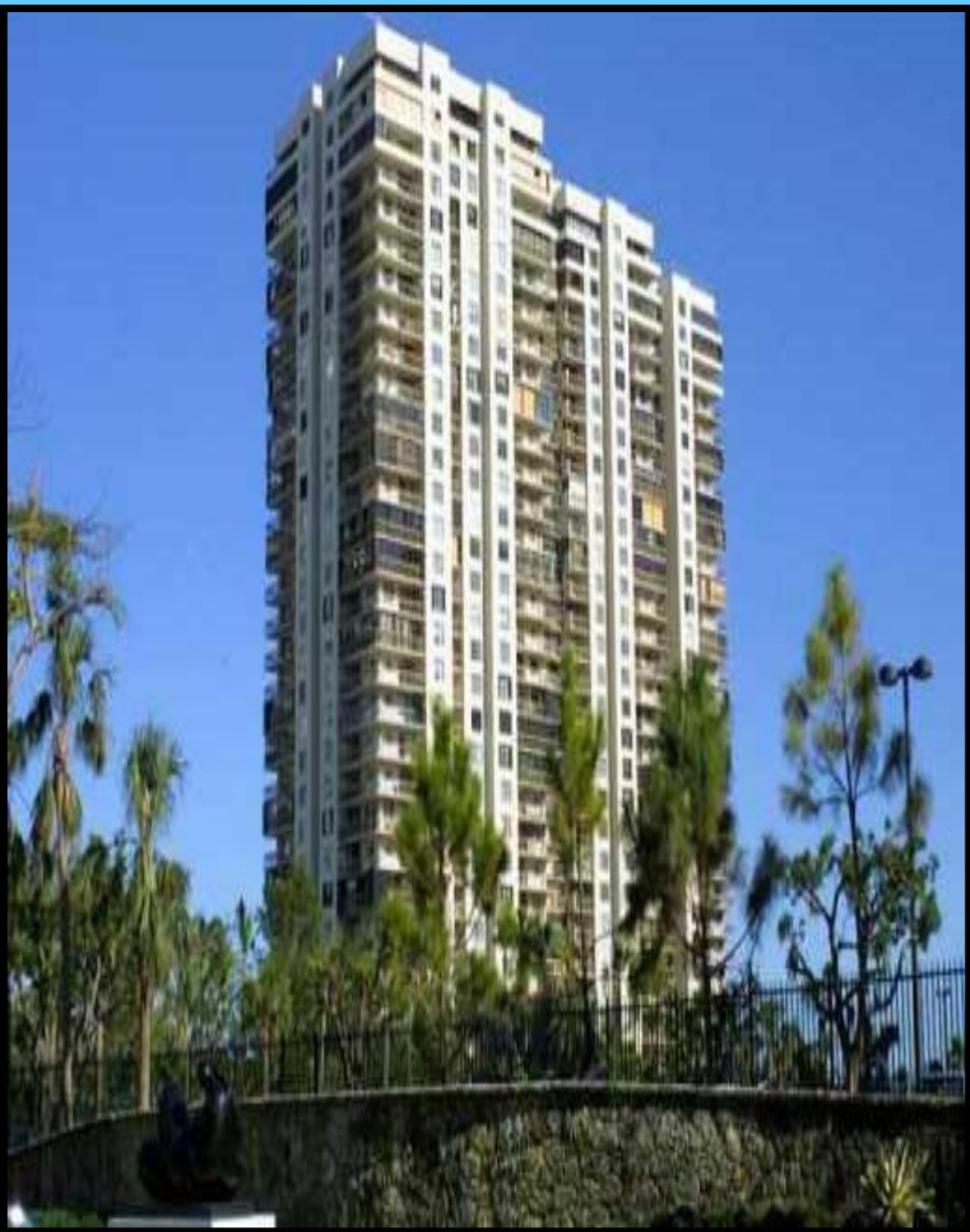
Typical High-rise older building
