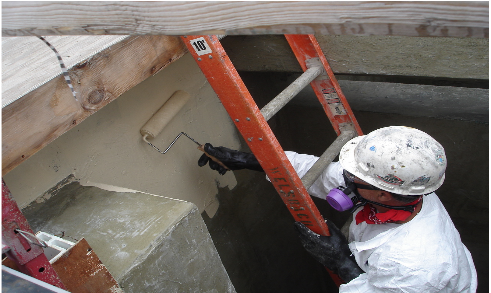
Hand rolling of final lining (sealer coat) on walls.
