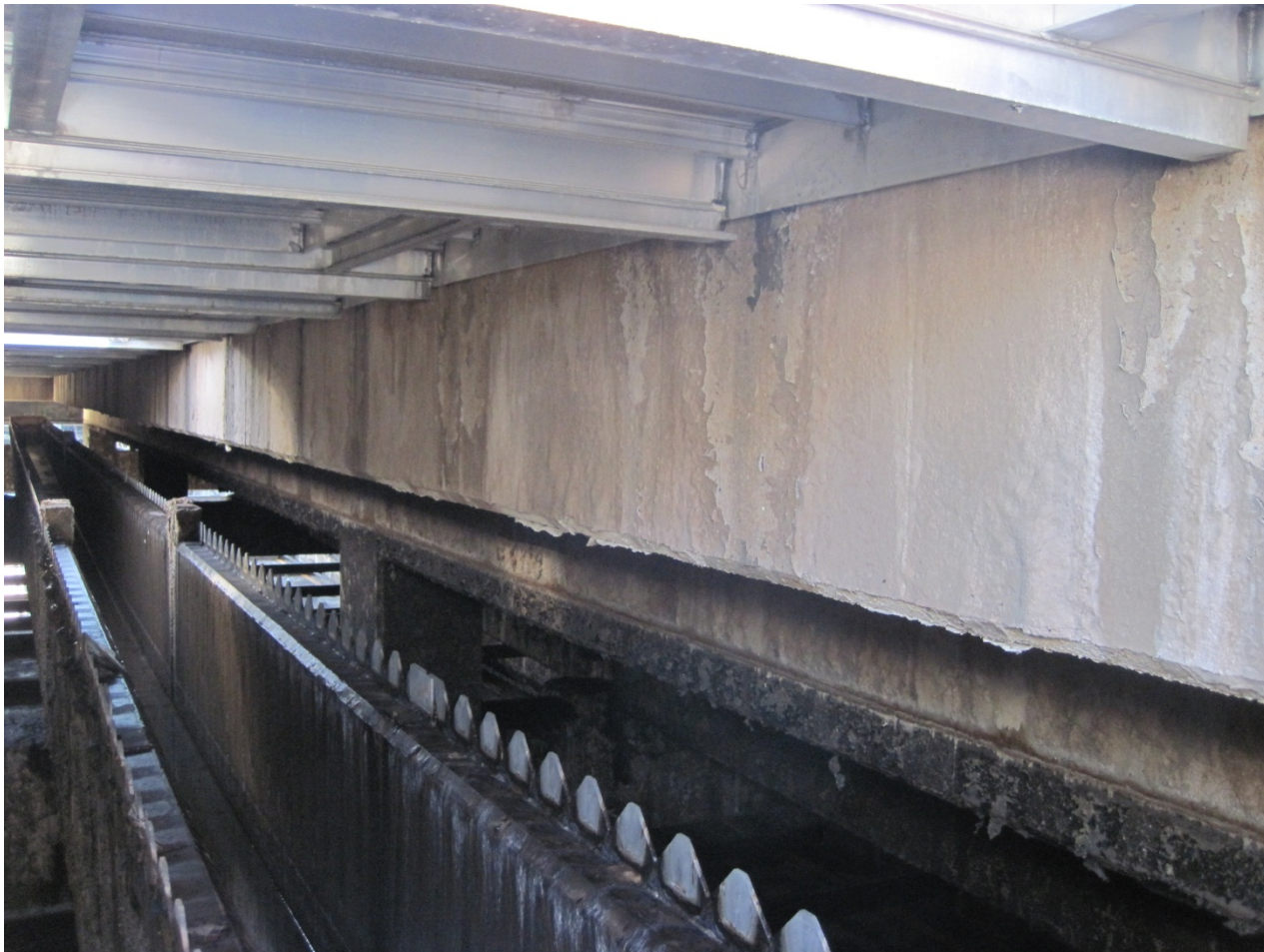
Concrete Walkway/Beam Over Covered Tank
