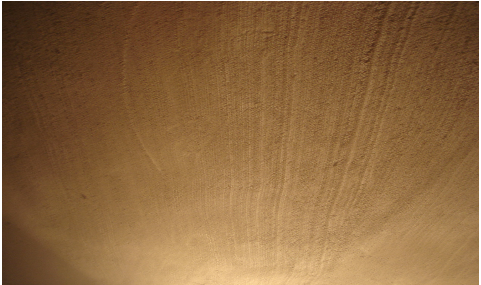
Underlayment with broom finish.
