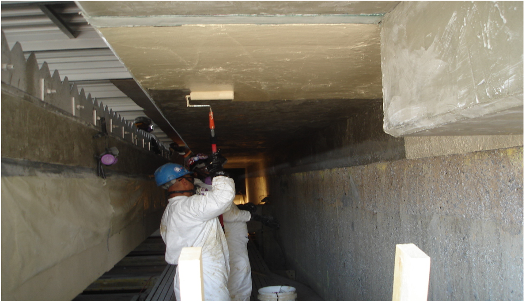
Application of final lining (sealer coat) on ceiling.
