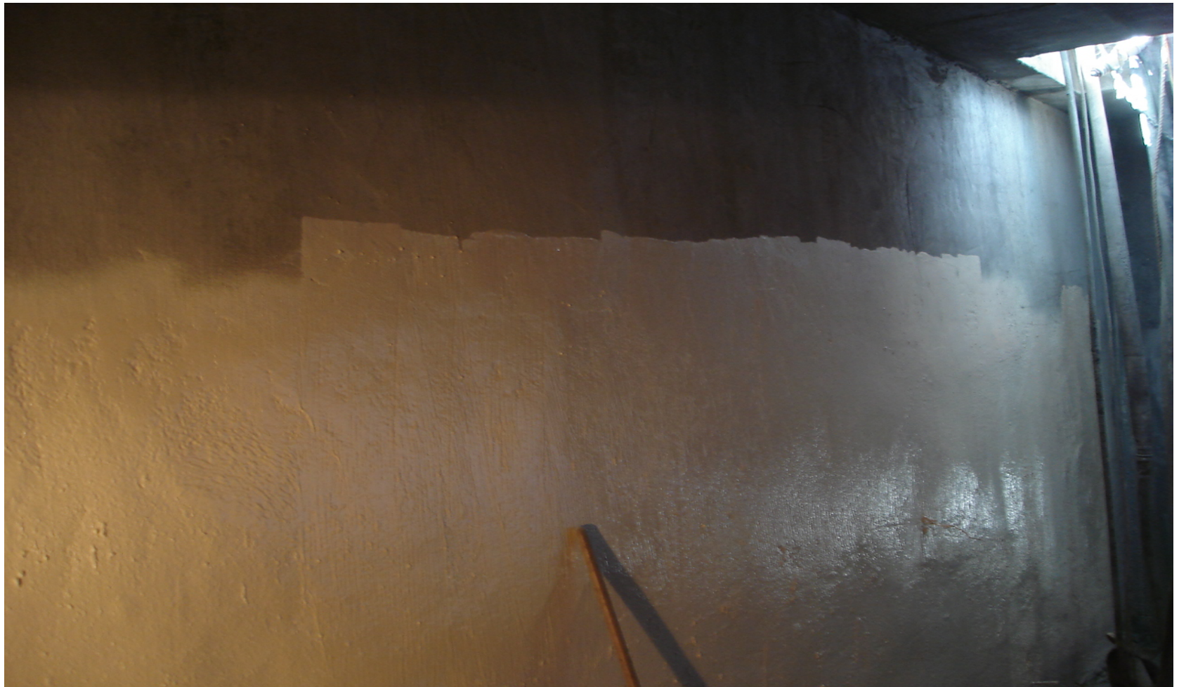
Partial coating of final lining (sealer coat).
