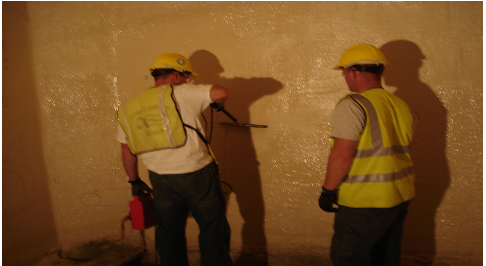
Spark testing to detect defects and pinholes in sealer coating.
