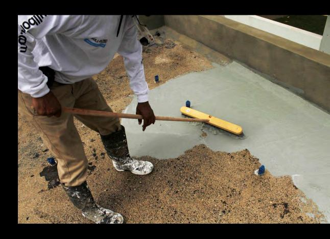
Thin cementicious mortar mix with latex to renew Concrete Surface
