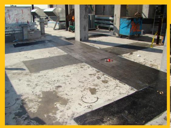
Carbon fiber fabrics bonded to roof slab to carry additional loads
