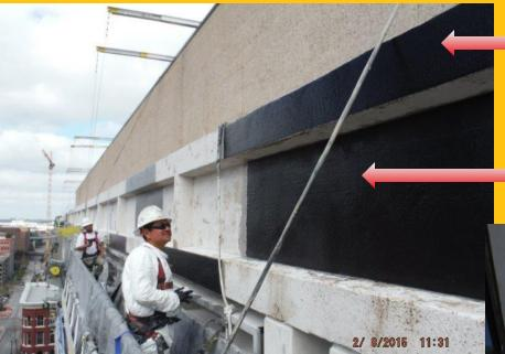
**Uni-directional CFRP fabric**
