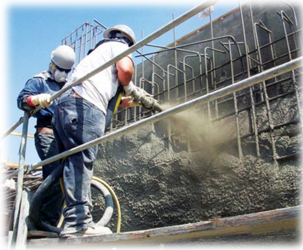
Traditional Shotcrete Repair
