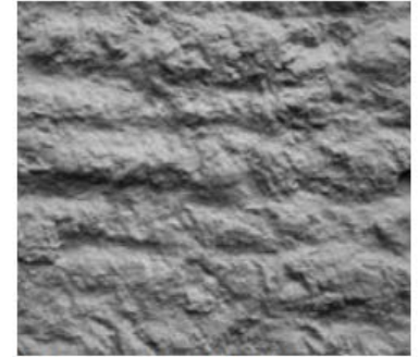
Fig. 6.9: CSP 9 (heavy scarification— rotomilled)
