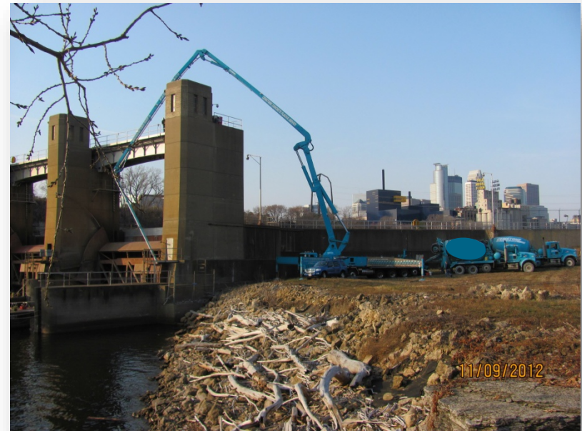
Concrete Placement - Gate Bay One, November 9 th 2012
