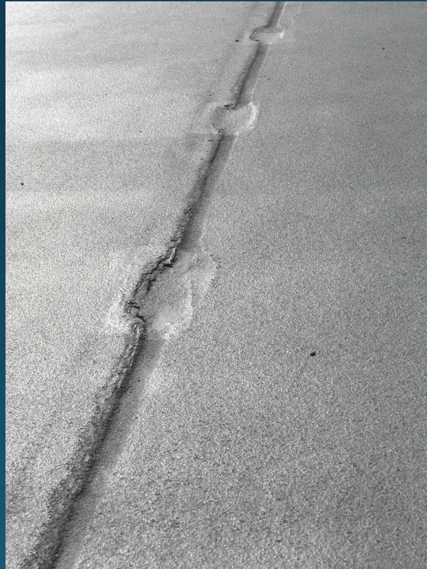
Ridges at weld pockets
