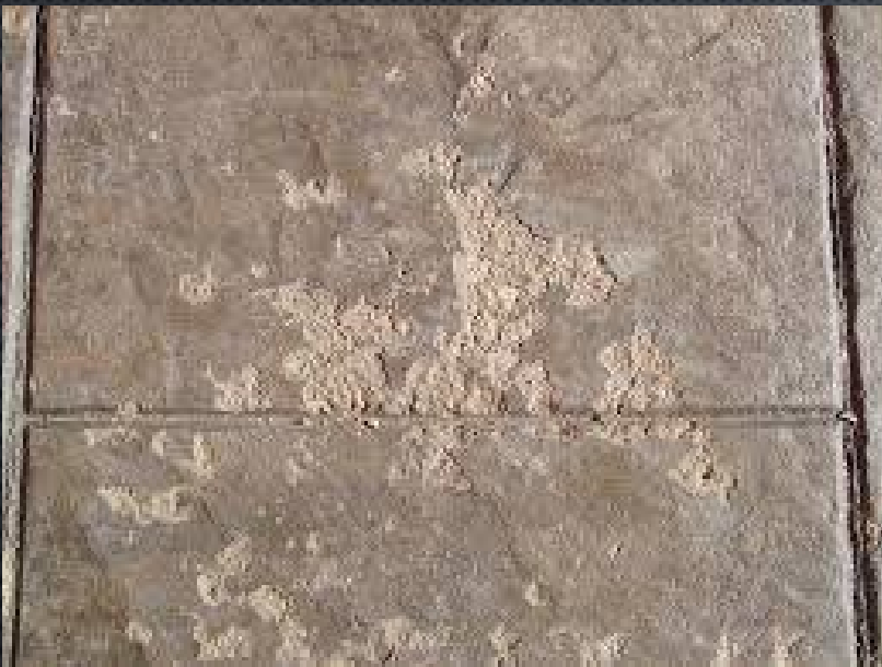
CONCRETE SCALING
