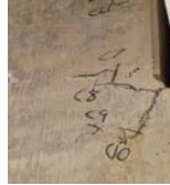
7.6.6 Repair geometry—Configuration of repairs shall consider the potential for stress concentrations and cracking in both the existing structure and the repair area.
