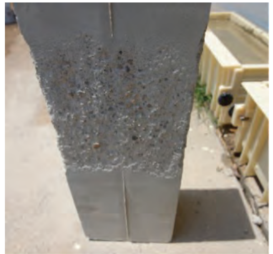
Fig. 1: Concrete pillar prepared to an ICRI CSP 5 in the test area
