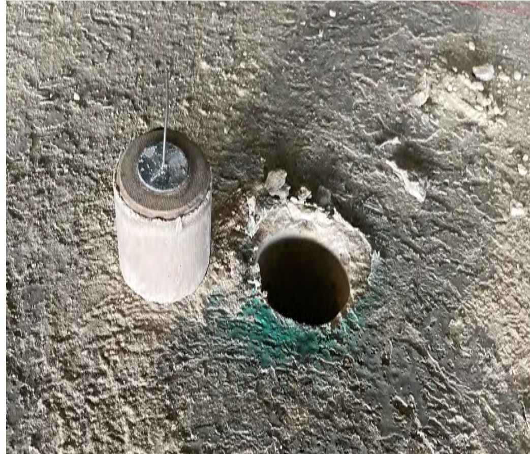
Type 2A Embedded Anode Next to Drilled Hole
