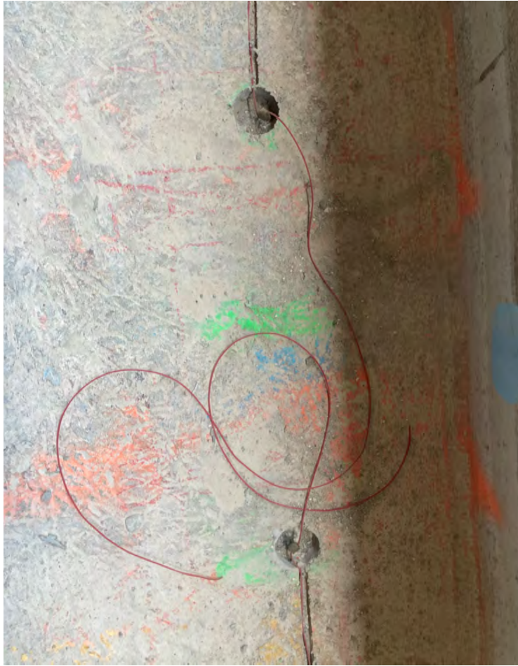
Two Series Of Anodes Ready to be tied to steel
