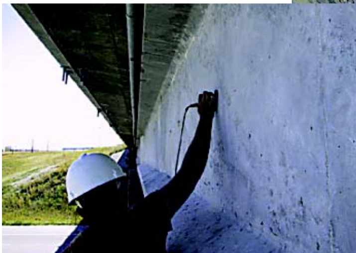
(b) UPV source on the east side of the east girder
