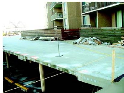
Slab and edge repairs complete
