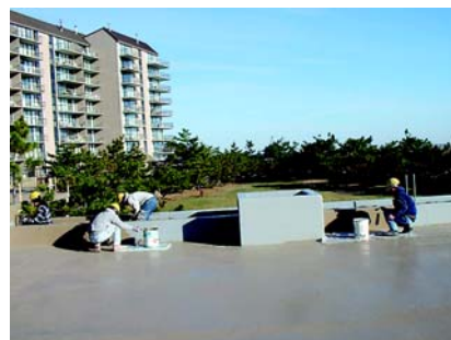
Applying urethane coating
