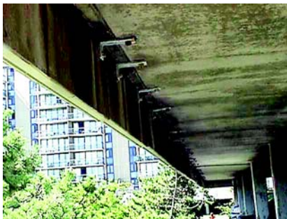
Bottom view of through-bolted angles
