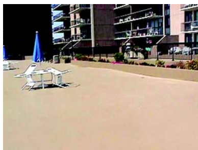
Promenade coated with planters finished
