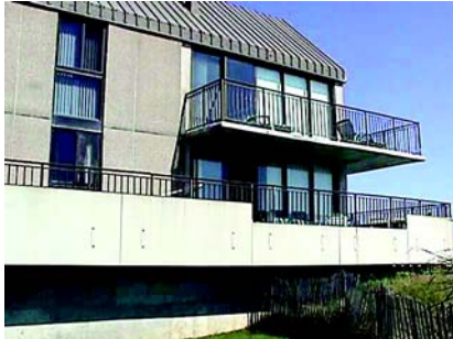
Promenade parapet panels
