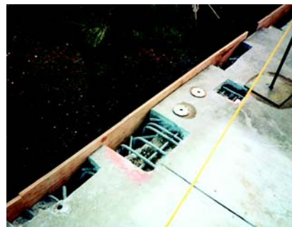
Parapet panels off and slab demolished
