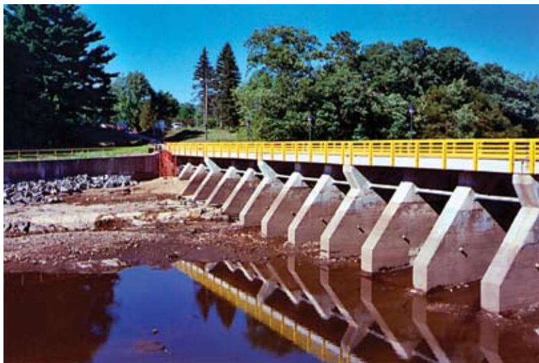
Completed guardlock bridge deck replacement (9/12/02).
