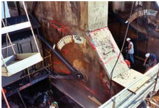
Gated section repairs in progress (9/5/02).
