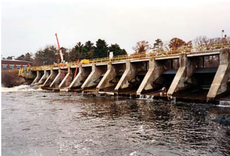
Completed gated section repairs (11/18/02).
