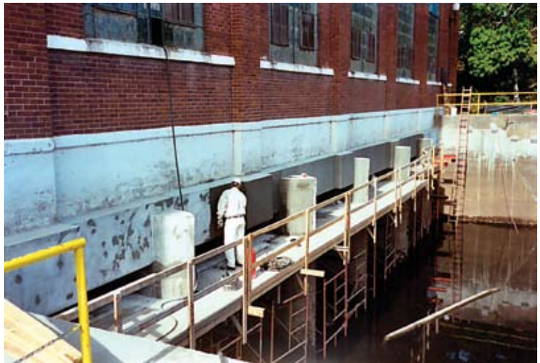
Completed powerhouse support beam repair (10/16/02).
