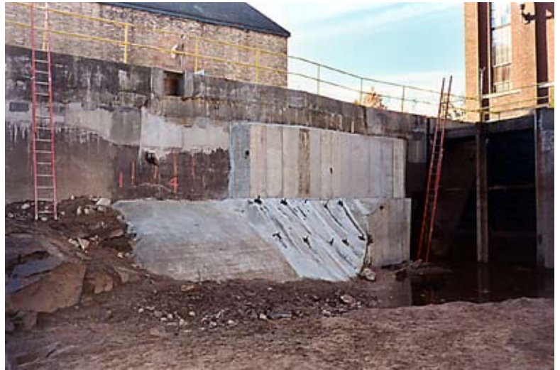
Completed SE forebay wall rock-anchored buttress wall repair (11/8/02).
