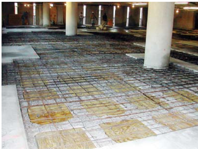
(Above and below) Large repair areas in the waffle slab portion of the garage prior to the placement of the new concrete. The wood forms are the bottom portion of the dome area of the waffle slab.
