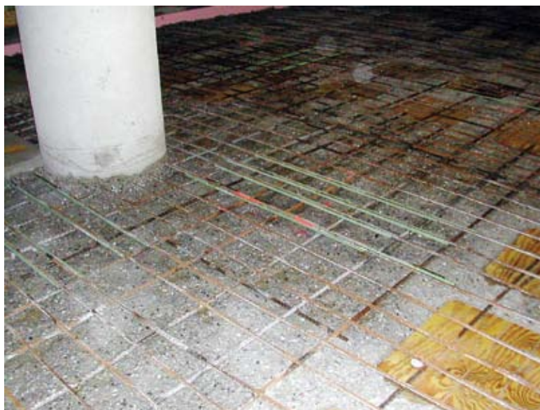
(Above and below) Large repair areas in the waffle slab portion of the garage prior to the placement of the new concrete. The wood forms are the bottom portion of the dome area of the waffle slab.
