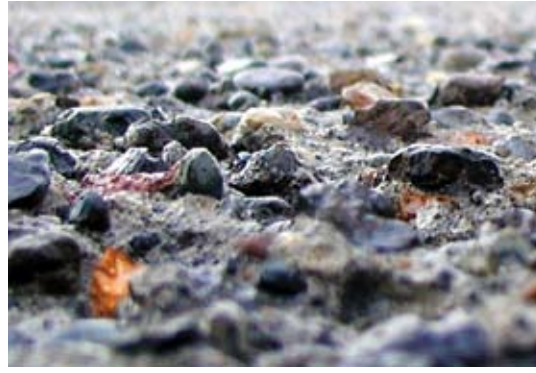
Fig. 4: Surface preparation using hydrodemolition. Exposed coarse aggregate improves bonding
