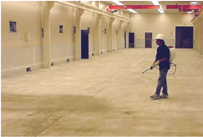
Fig. 2: Spray-applied reactive penetrants combine with alkalis within the concrete, reducing the pH and permeability to moisture vapor (photo courtesy of SINAK Corp.)
