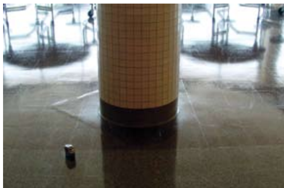
Fig. 5: Reverse warping around isolated diamond blockout at column footing
