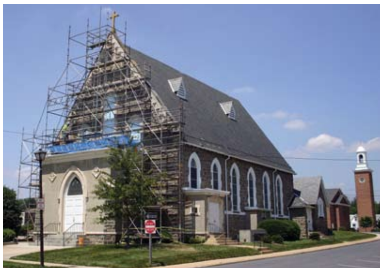
Fig. 5: Scaffolding erected to help ensure safety
