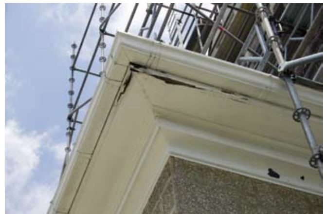
Fig. 2: Pre-existing wood trim condition
