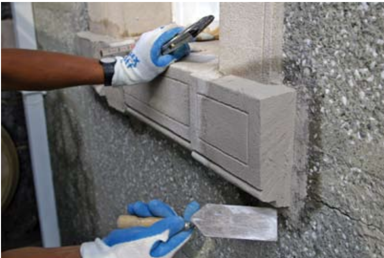
Fig. 6: Repaired sill prior to coating application
