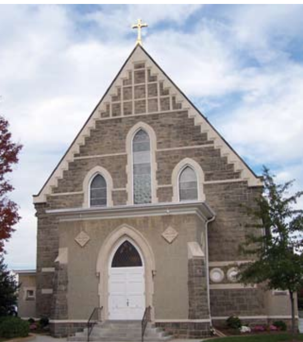
Fig. 8: Completed front façade of St. Mark's Church
