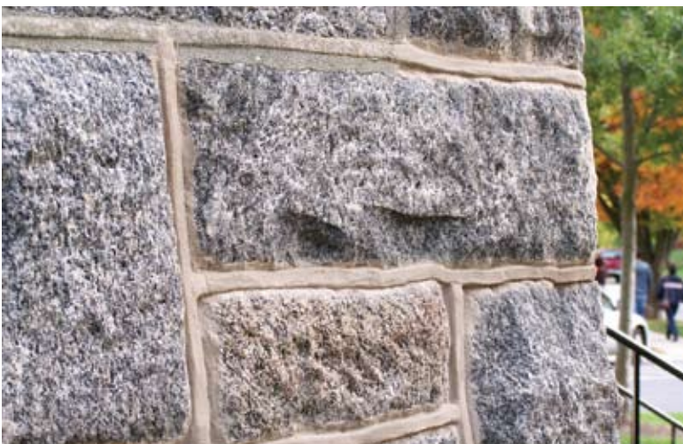
Fig. 7: Repaired pointed mortar joints with high-grade mortar material
