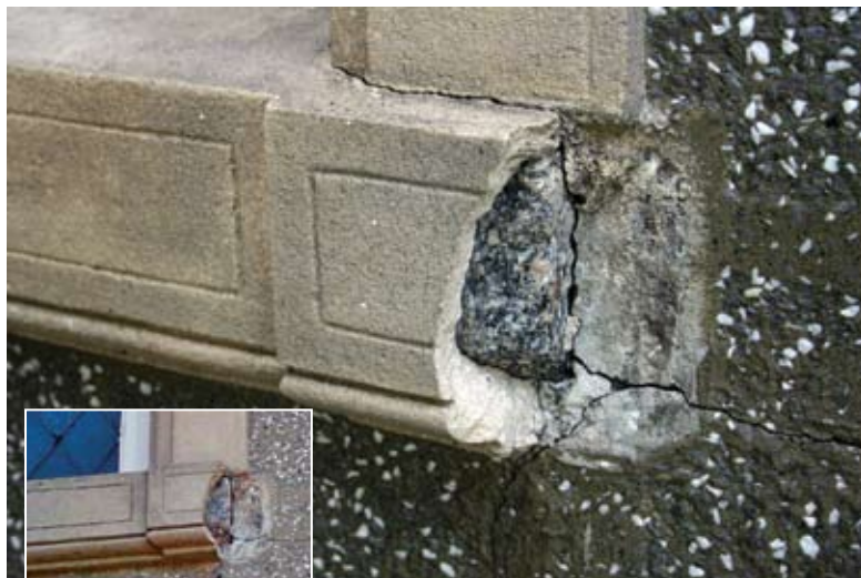
Fig. 3: Typical existing condition at faux limestone sill
