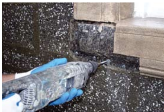
Fig. 4: Pin installation for faux limestone repair
