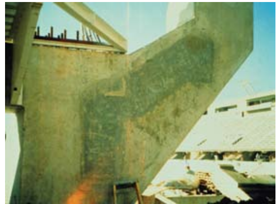
Cementitious concrete repair mortar applications
