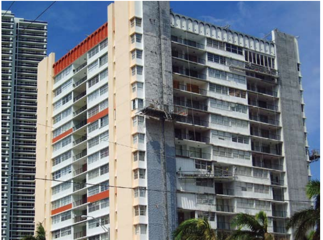
HEK platform used to execute repair work
