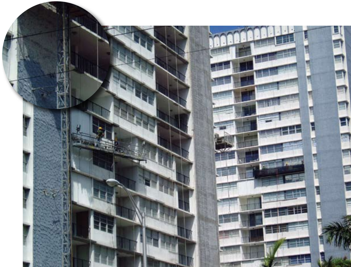
Removal of old stucco
