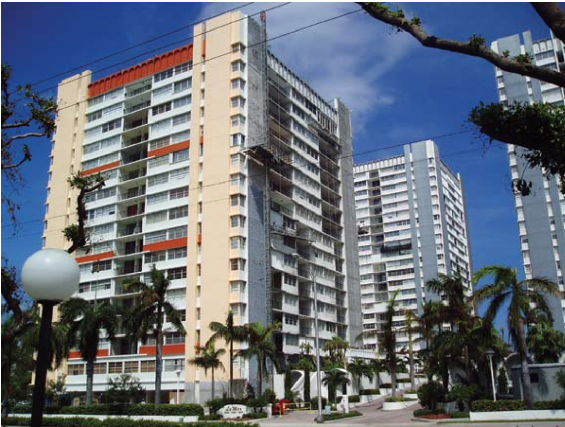
One side complete façade repaired with new appearance
