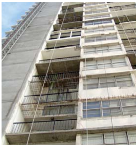
Repairing deteriorated balconies
