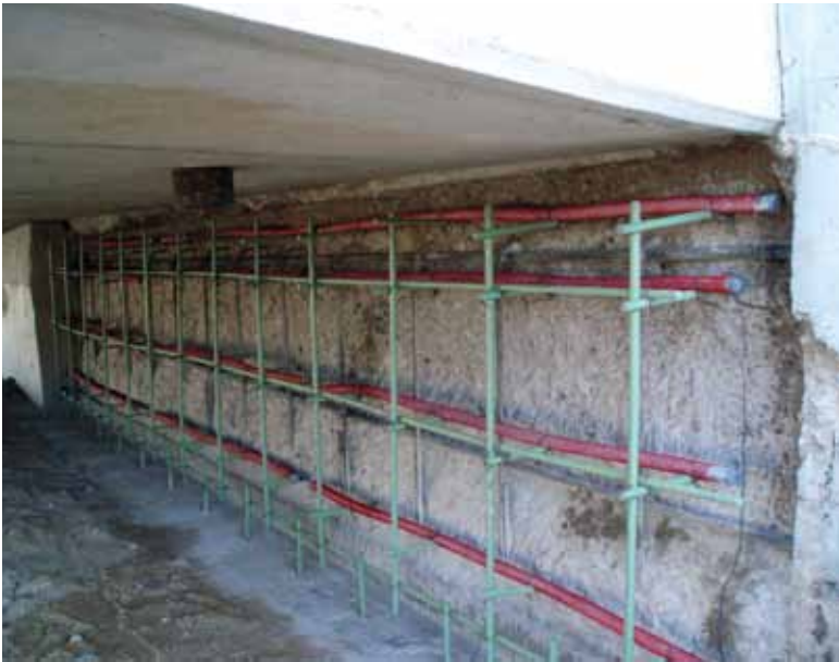
Distributed galvanic anodes used in galvanic encasement repair of bridge abutment
