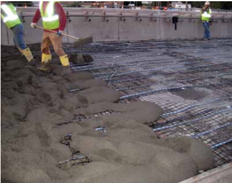
Distributed galvanic anodes used in conjunction with bridge deck overlay
