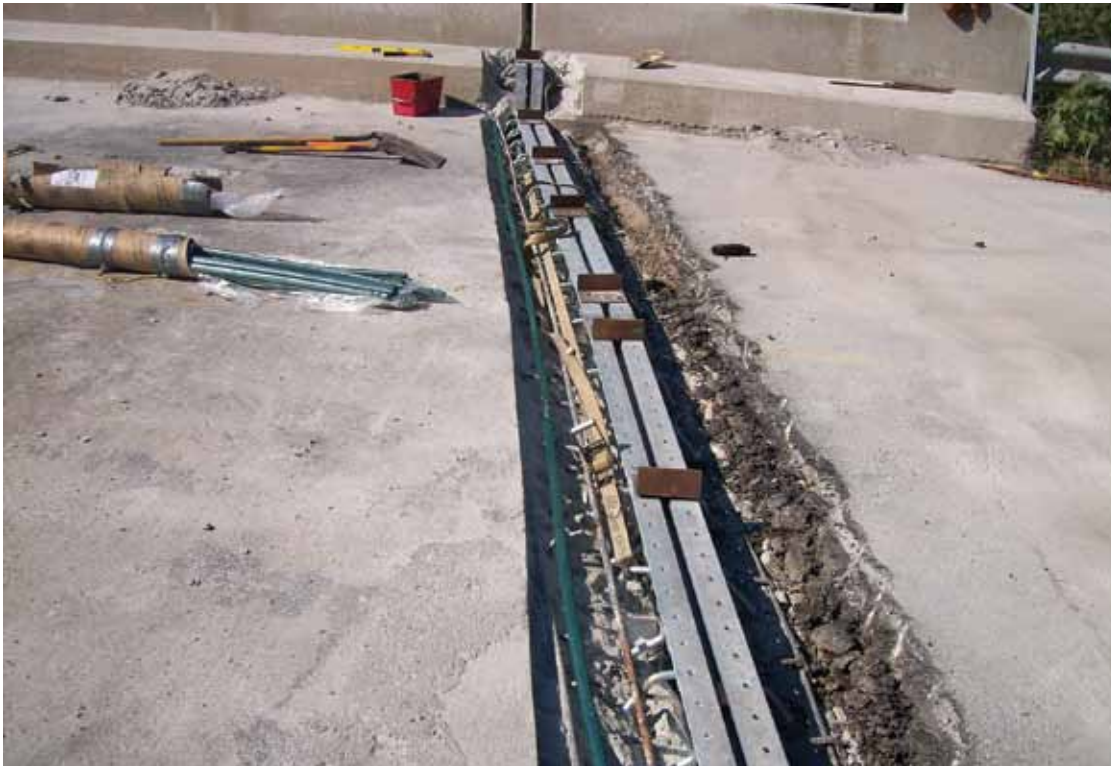
Distributed galvanic anode installed along expansion joint repair
